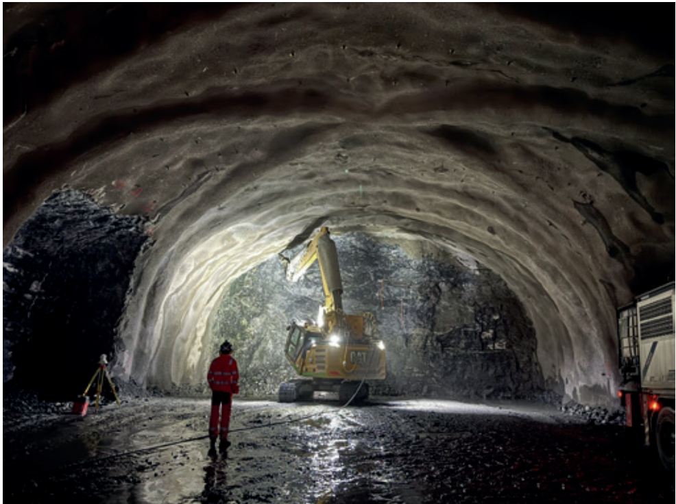
Figur 15 Tetterresultater observert i tunnel under driving.
