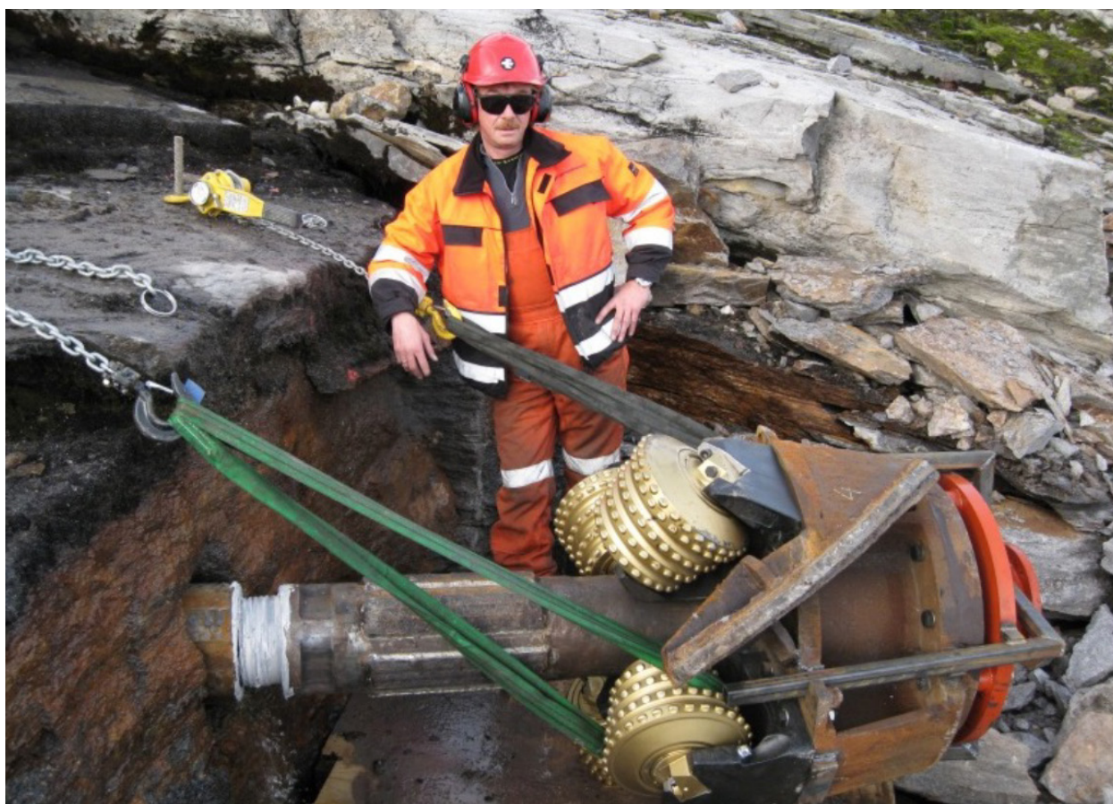
Figure 2.7. Raise drilling. Ready for reaming the shaft (Photo: Bård Skatvold).
