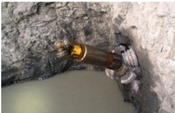
Figure 2.8. Norhard breakthrough with pilot hole on Grytendal project (NGK, 2019).
