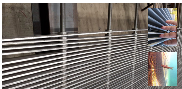
Figure 3.3. The grid with small slits in front of the water intake. (Photos: Voss Energy and Multiconsult).
