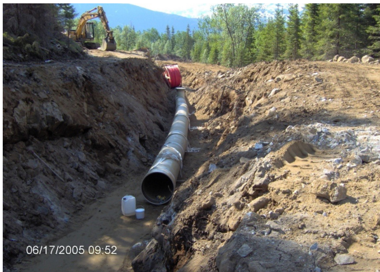
Figure 2.1. Installation of penstock in ditch (Photo: Werner Stefanussen).
