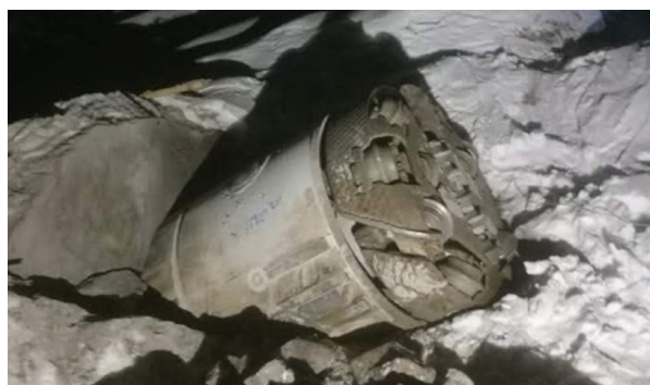
Figure 5.2. Breakthrough at Holen SHEPP (Photo: Hardanger Maskin AS).
