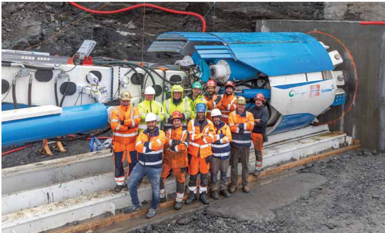
TBM klar for borestart, Salvasskardelva. Foto: Kalle Punsvik/ The Robbins Company
