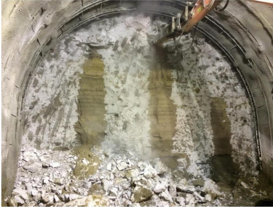
Figure 3: Example of face and perimeter stabilization of soil tunnel including face support columns, Trevi SpA
