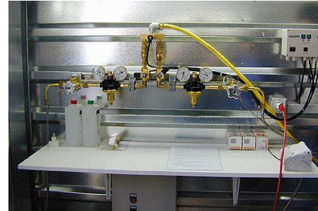
View into the control room
