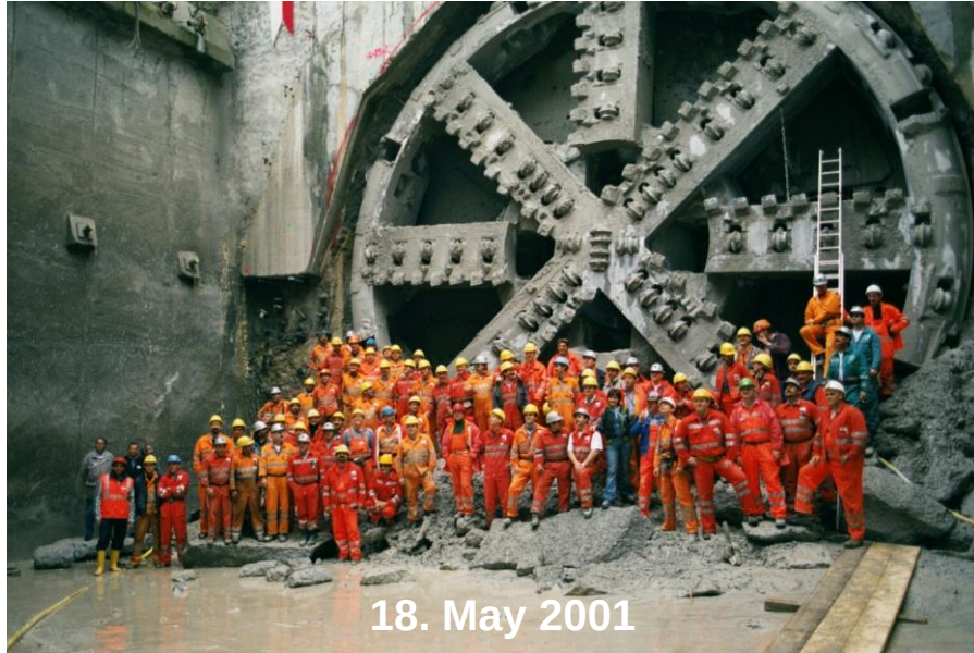
Breakthrough Zimmerberg Basetunnel in Zürich (Mixshield)
