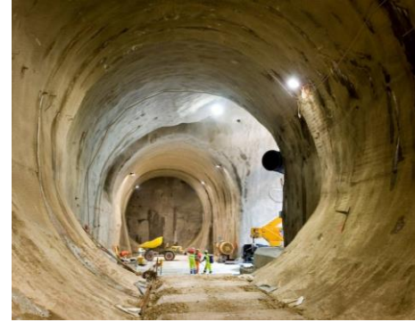
Loose soil excavation Main tunnel
