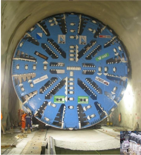
Mixshield TBM Main tunnel
