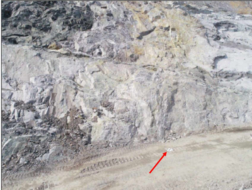
Fig 5. An example of a ground control point at the toe of a slope (profile 15300).
