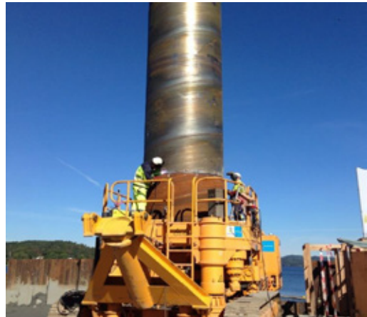
Figur 13: RDM 2000 Casing Rotator
