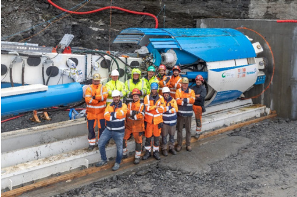
Figure 8 TBM ready to start boring Sallvasskarelva (Photo: Kalle Punsvik)
