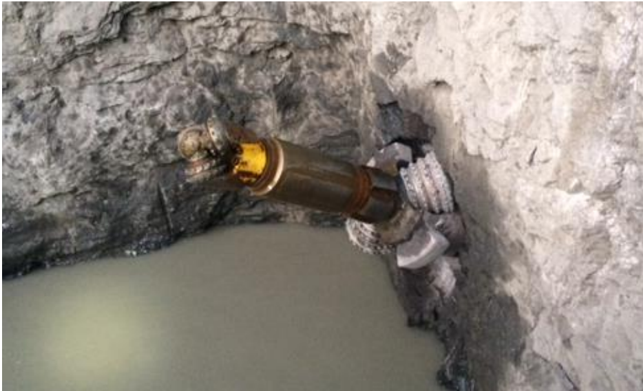
Figure 4 Norhard breakthrough with pilot hole on Grytendal project (NGK, 2019)
