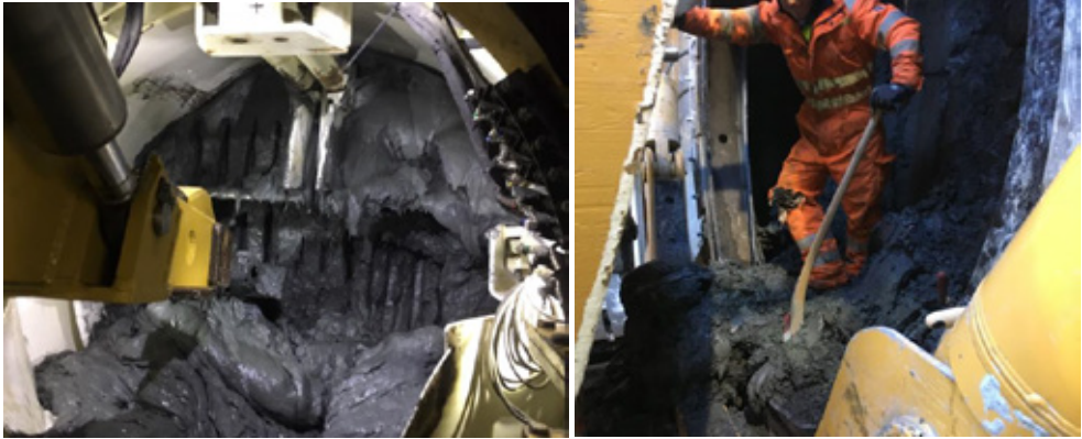
Figur 21: Graving i front
