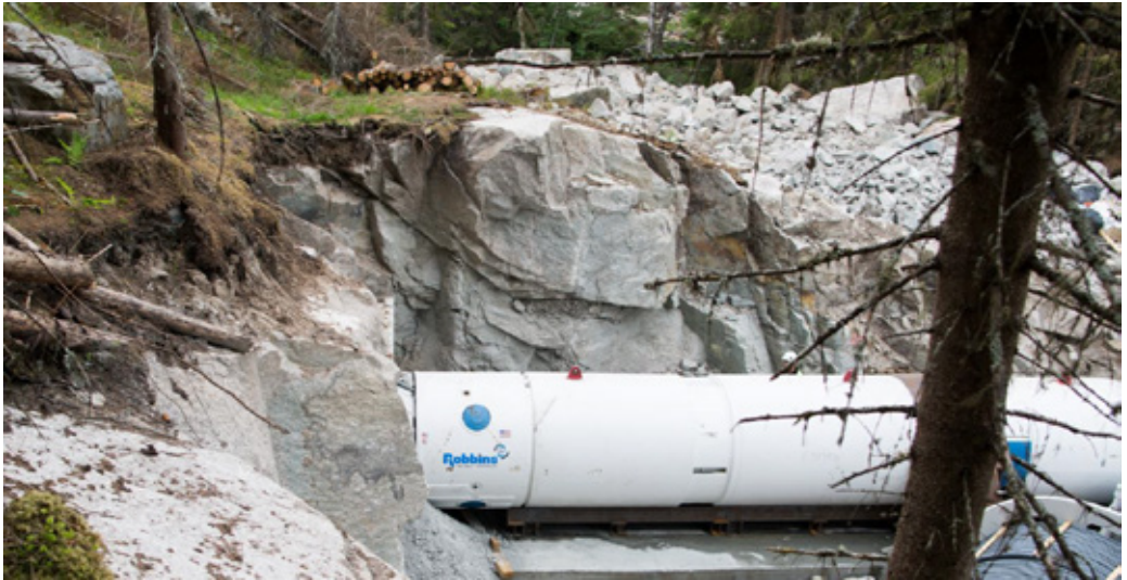
Figure 6 TBM at Holen HEP (Photo: Endre Hilleren)
