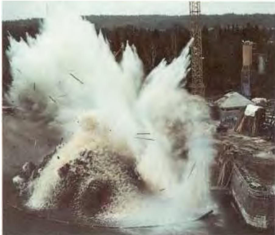
**Before and during blasting of the cofferdam, at Solbergfoss hydropower plant. The cofferdam is mostly formed by rock masses, with a distance from the intake structure of 5-10 meters (Oslo Lysverker)**
