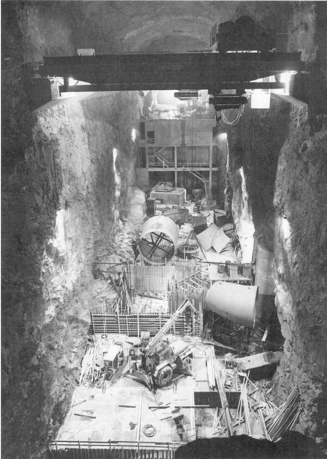
**The Alta underground powerhouse during installation of the draft tubes.**
