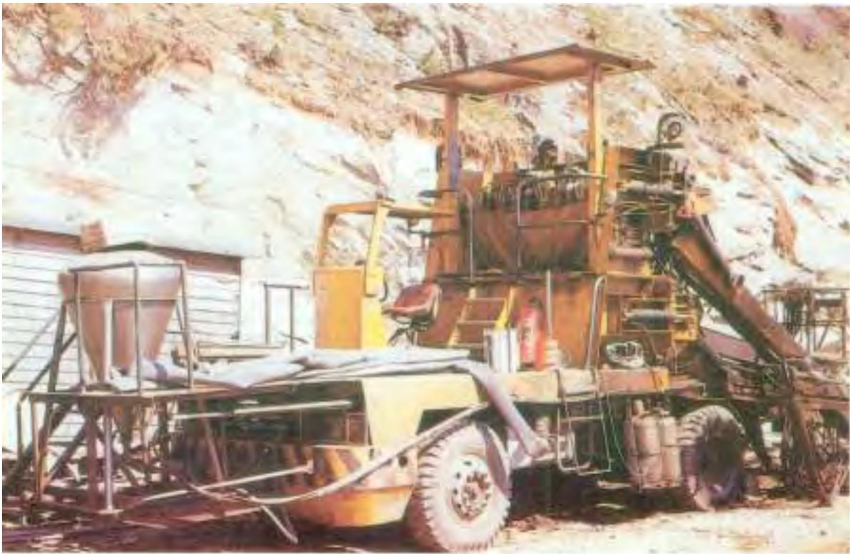
*Old modern drilling jumbo with ANFO charging equipment built in 1974 (Norwegian Geotechnical Institute)*
