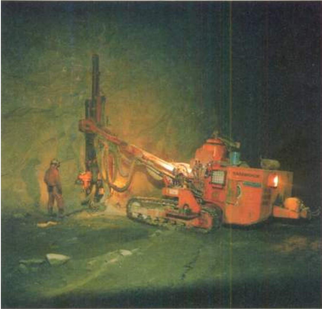
**Drilling of blast holes for benching of an underground power station (Berdal)**
