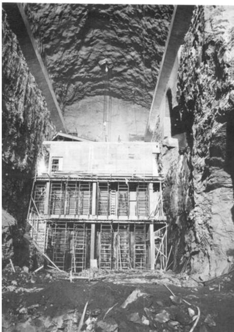
*Installation work in the Alta underground powerhouse. The span is 16 meters the height is 35 meters. (Photo: Ole M. Rapp.)*
