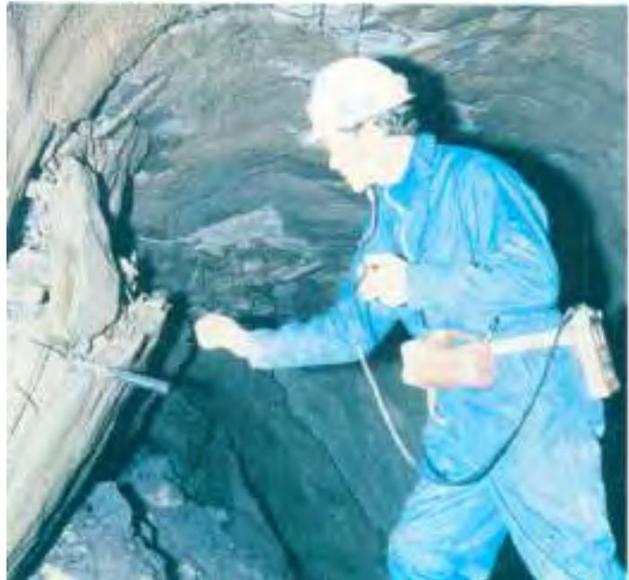
Rock slide in a water tunnel. An engineering geologist inspecting the failure caused by insufficient rock support of a weakness zone containing swelling clay. (Norwegian Geotechnical Institute.)
