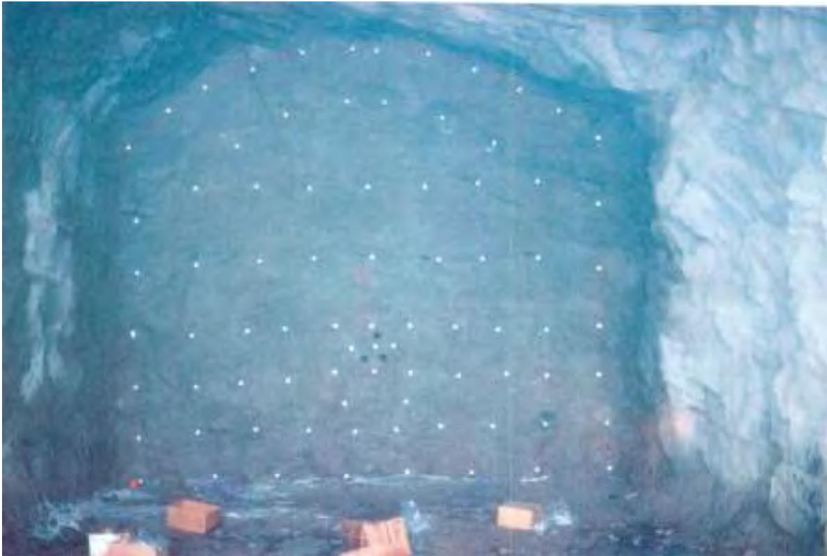
*Drilling pattern in a 40m<sup>2</sup> tunnel drilled with a computer-controlled jumbo (Norwegian Geotechnical Institute)*
