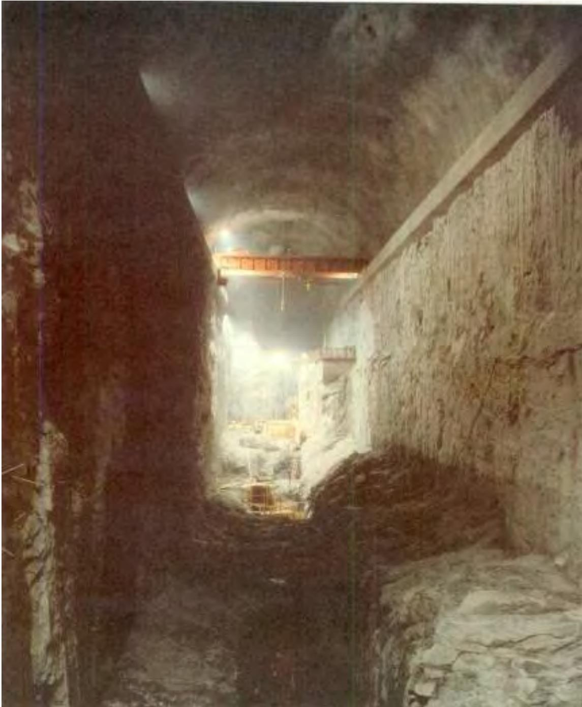
Saurdal underground hydropower station after excavation shown prior to installation work. Norway has nearly 200 underground hydropower stations in rock, a design with many advantages as described in chapter 12.
