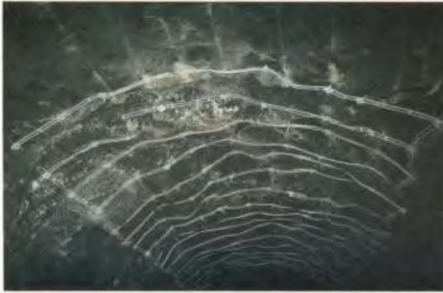
*Rock bolts, steel straps and net, in a tunnel subjected to heavy rock burst.
