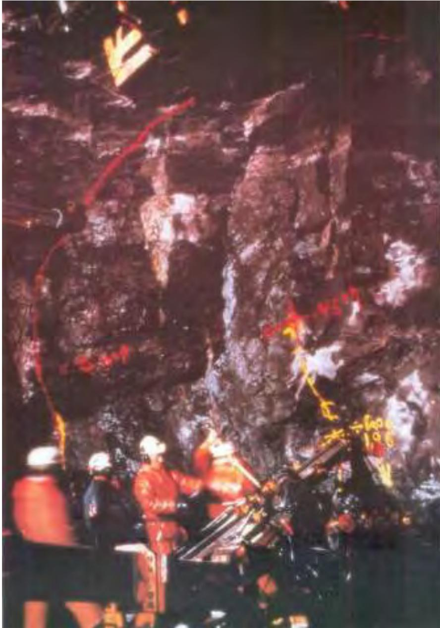
Photo 17.2 Drilling of grout holes to seal a water leakage in front of tunnel face. (O. Aasen)
