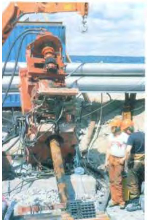
*Photo 16.2 Drilling of the pilot hole (Entreprenørservice A/S)*
