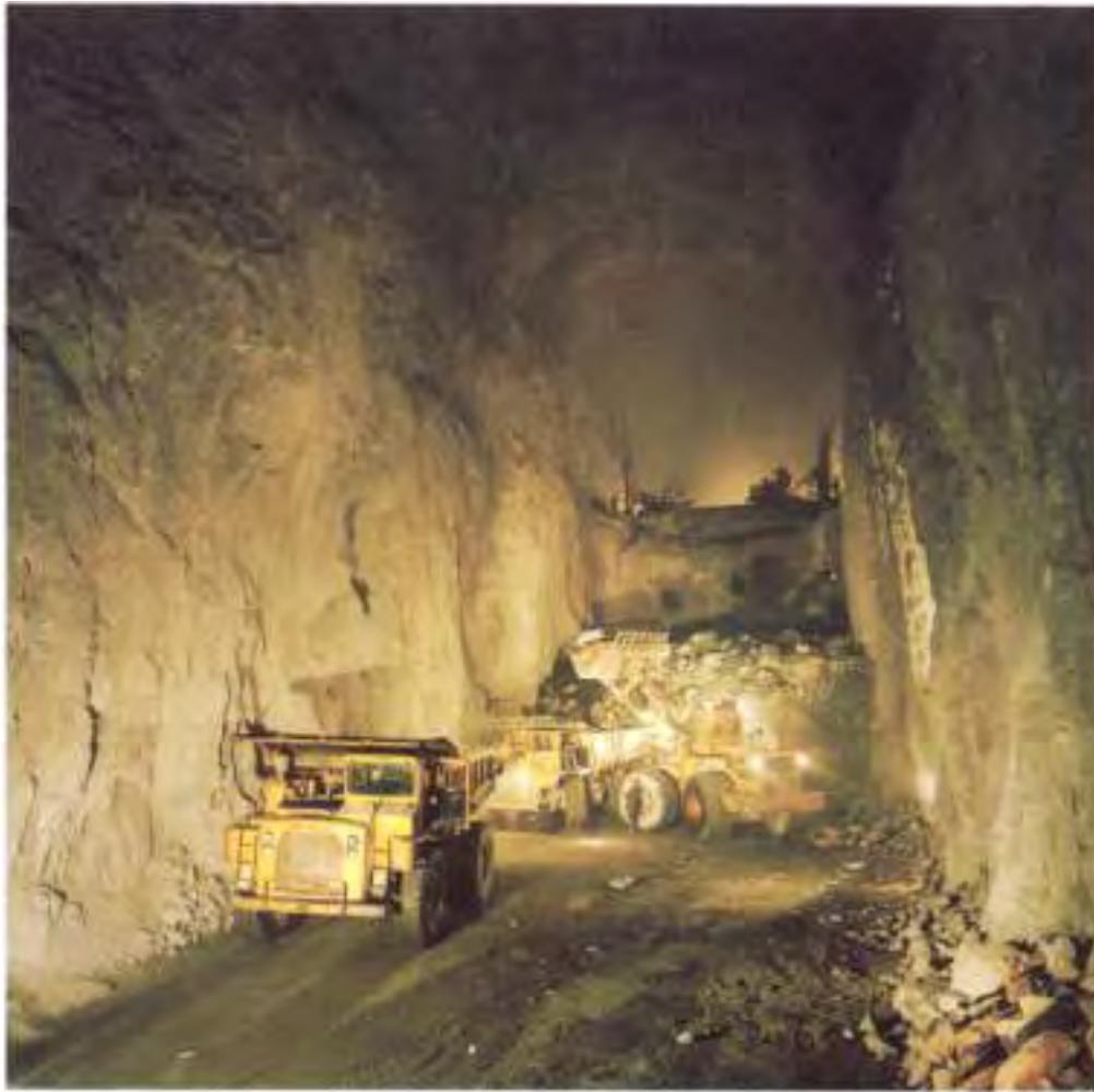
**An underground oil storage cavern. These caverns with cross section  $530 \text{ m}^2$  was excavated in four stages: Top heading and three benches (Berdal)**
