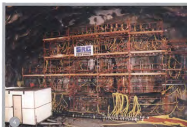
Ground freezing in the Oslofjord Tunnel. Photo Eirik Øvstedal
