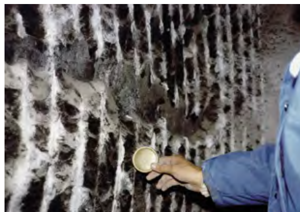
Figure 3. Void in the tunnel face created from a plane of weakness (3).
