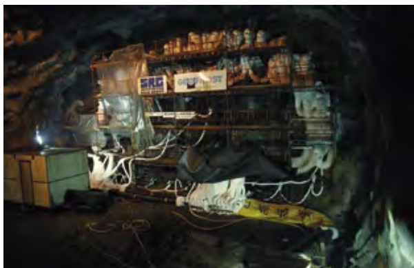
Fig. 3: Frozen contour with freezing pipes appearing as cone is decreasing.
