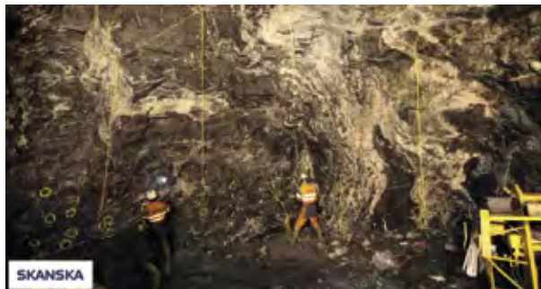
Picture 4 Tie in sequences. Exel tube bunches (upto 20 tubes) hooked up with detonating cord around the face.
