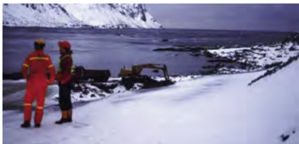
Fig.1 Excavation for the portal of the Nappstraumen sub sea road tunnel
