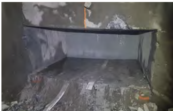
Figure 18. Breakthrough to existing intake tunnel with wire sawing.
