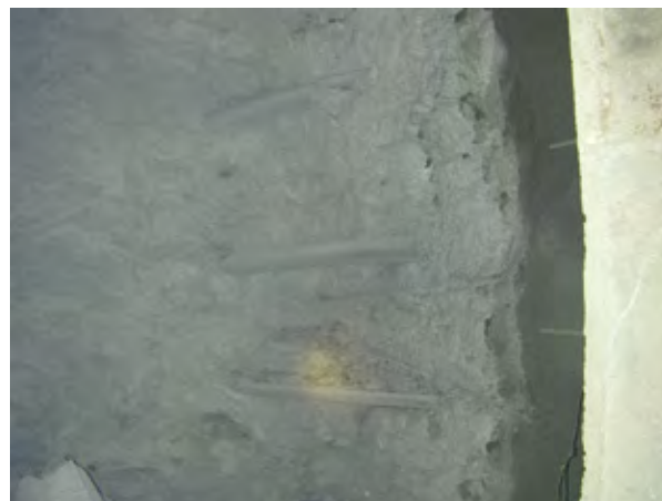
Fig. 2: Frozen glaciofluvial material after blasting.
