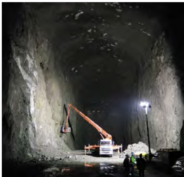
Photo 2. Lorry-mounted inspection platform for mapping and installation of rock support. Photo by FSA, Multiconsult.
