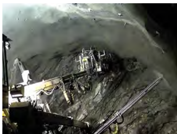
Image 20 – Installation of the CT-Bolt®
