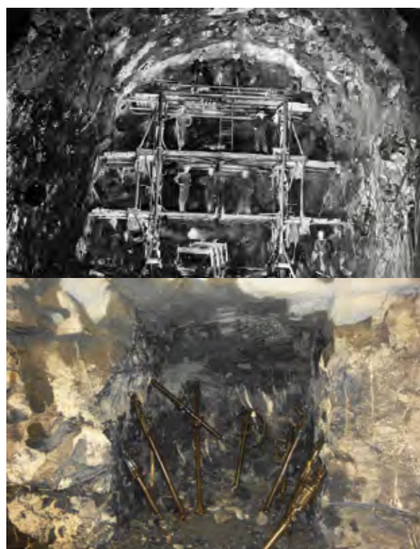
Tunnelers at work at the tunnel face, Tokke Hydropower Project, and drilling equipment from early 1950'ies
