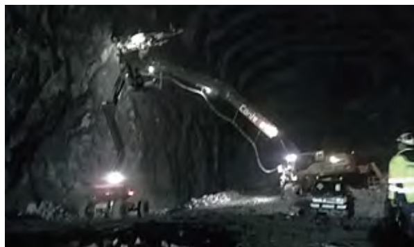
Photo 5. Installation of rock support in wall by drilling with long stick excavator with hydraulic hammer. Bolt installation is carried out by operator in a separate lifting platform. Photo by FSA, Multiconsult.
