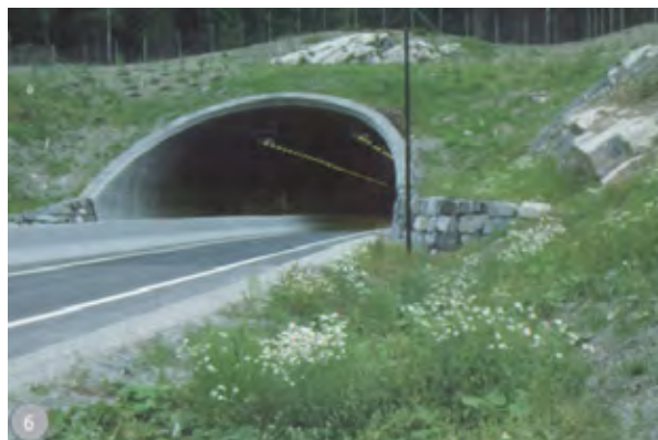
A good tunnel portal according to requirements in the 1990s. Today, requirements as regards traffic safety in tunnel openings are more rigorous, especially when it comes to guard-rails, funnel design and adaptation to the terrain. Photo Eirik Øvstedal
