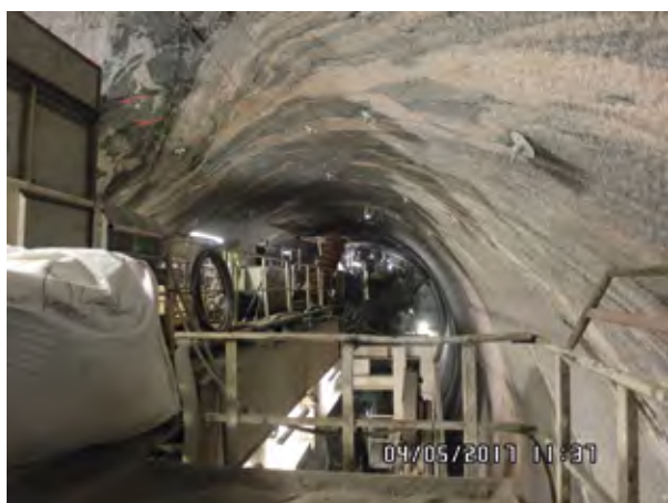
The Ulriken TBM tunnel. The rock mass consists mainly of Gneisses. Photo: Bane NOR
