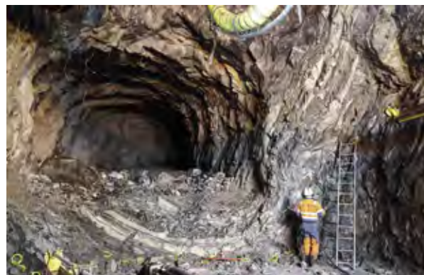
Figure 16. Charging the next round in the access to the intake chamber.
