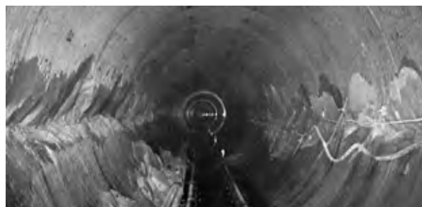
Figure 10. “Dog-earing” in sandstone due to high vertical stresses in the Delivery Tunnel in Lesotho
