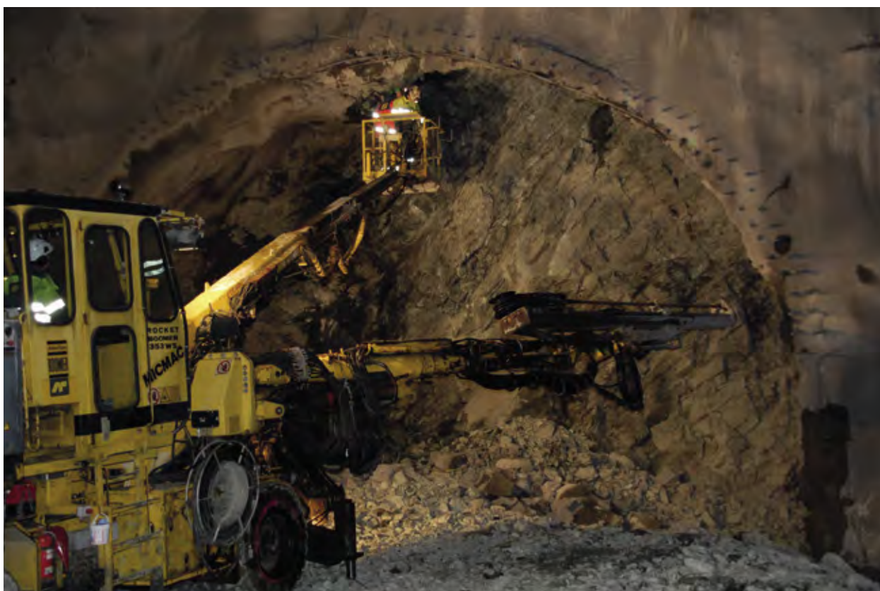
At this location the Engineering geologist and the Contractors Site manager together decided double spiling bolts, perform pre-injection to stabilize the rock formation, to blast the cross-section in two blasts and use reinforced shotcrete arches together with spiling c/c 2 meters.
