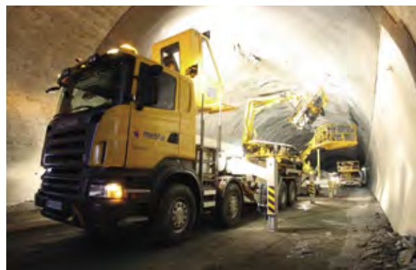
AMV 236-T Bolting rig used for drilling of bolts for membrane, PE foam and bolts for concrete elements.
