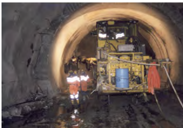
Fig. 7 Drill and blast excavation in difficult rock mass conditions in the Frøya tunnel where extensive shotcreting and concrete lining were required.
