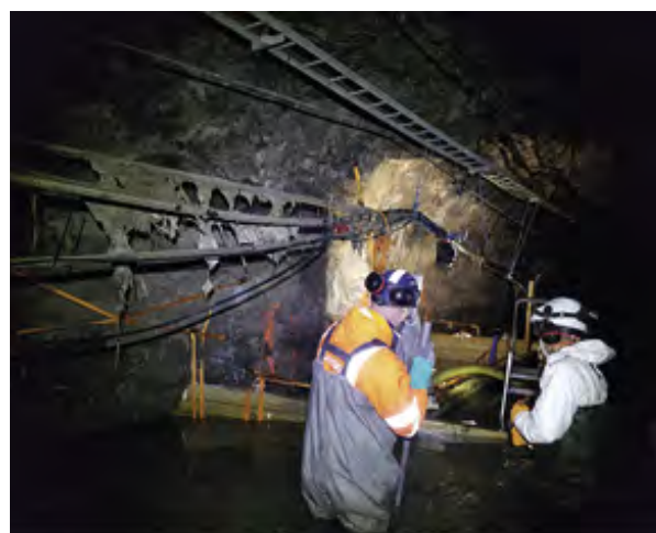
Figure 17. Preparing for breakthrough to the intake sewer tunnel – in full operation.
