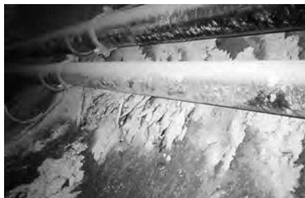
Figure 7. "Crazing" due to weathering in amygdaloidal basalts in the Transfer tunnel in Lesotho.
