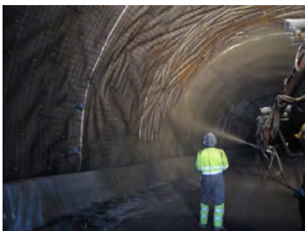
Shotcrete on insulation material. Photo Harald Buvik
