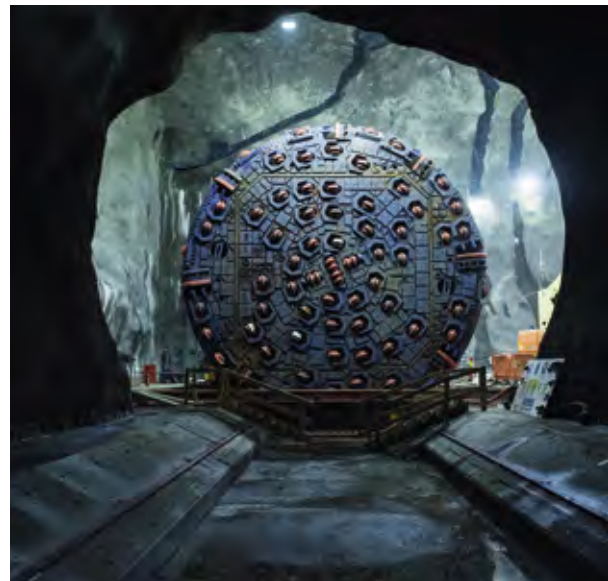
Figure 2: Launching of TBM S-982. Photo: Acciona-Ghella Joint Venture
