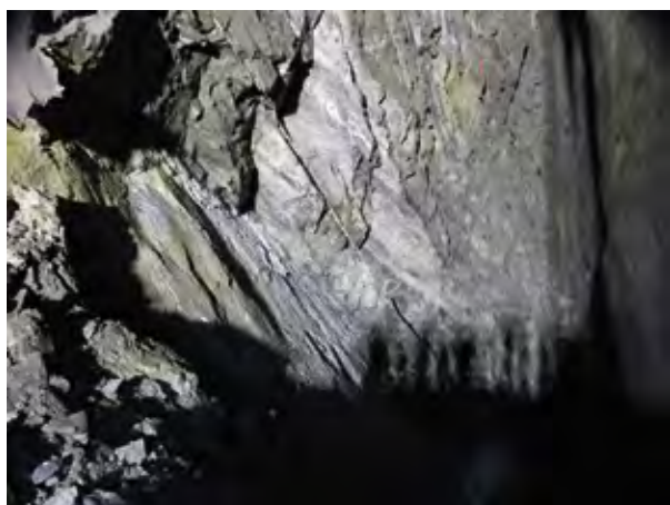
Photo 4. Close up photo of zone with infilling of swelling clay (light gray). Photo by FSA, Multiconsult.
