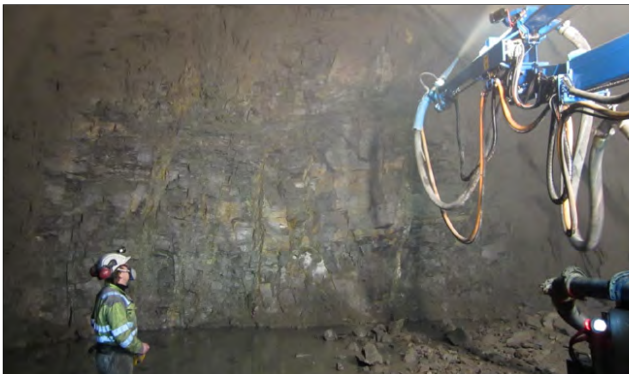
Figure 5: Spraying robot operated by remote control
