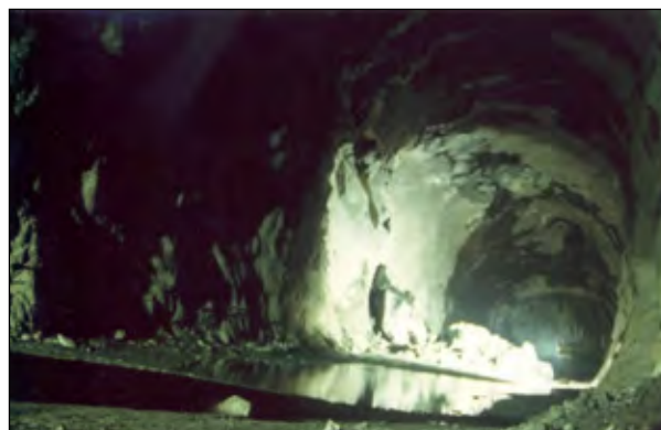
Figure 4. Examples of rock spalling (left) and rock burst (right) in deep-seated tunnels
