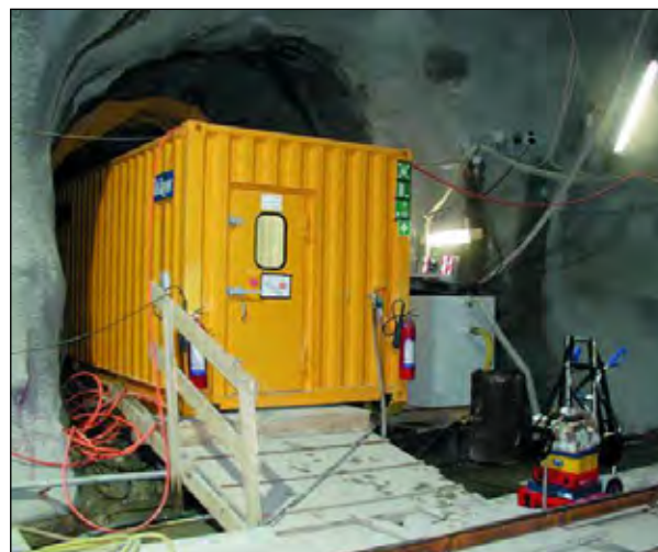
Figure 12.3: Rescue container with oxygen shall be placed maximum 500 m from face.
