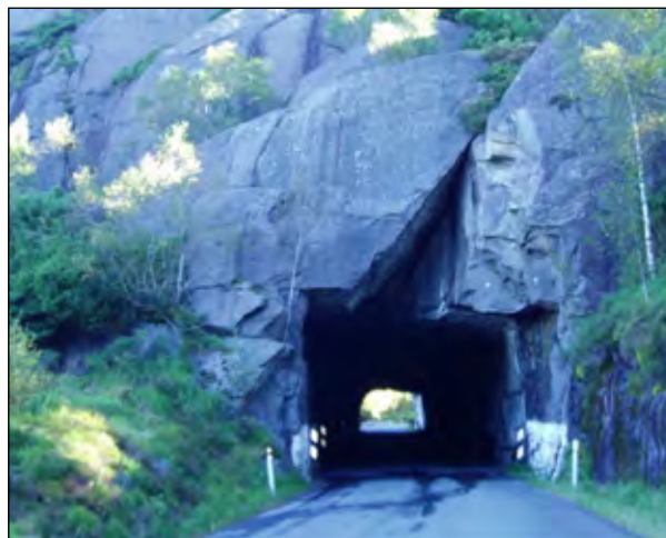
Figure 1. Example of instability caused by intersecting joints (old, low traffic road tunnel).
