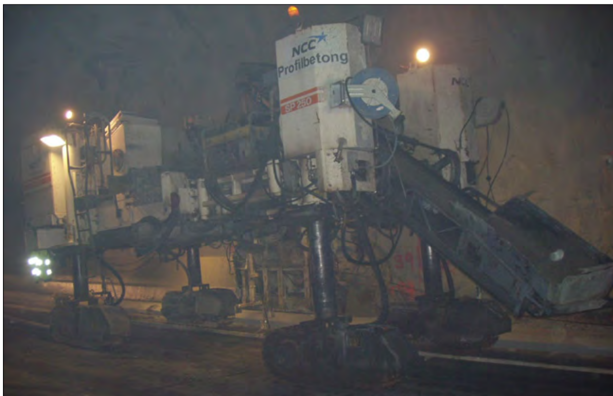
Figure 1: Concrete pouring of barriers
