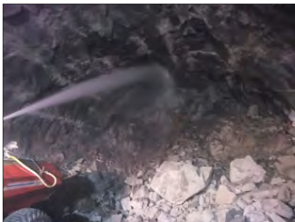
Figure 2: Watering a muck pile
