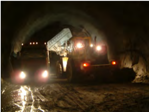
Figure 3: Loading at the face without generating dust
