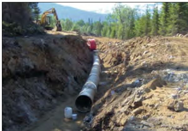
Figure 1. Installation of penstock in ditch
