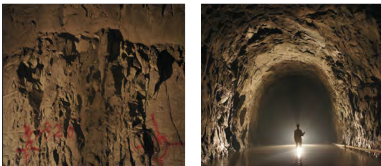
Figure 5 - Typical “Crushed zone” (left hand side) and “Extremely Good” (right hand side) rock mass conditions.
