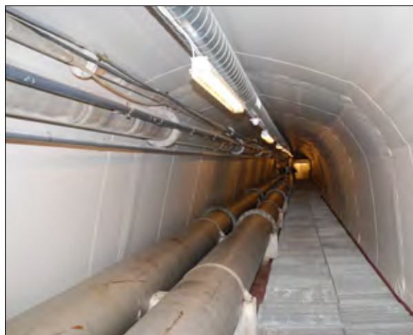
Figures 1 and 2: The picture to the left shows a typical situation in a pipe access tunnel where you have a wet and humid environment that gives corrosion problems to steel pipes and electrical equipment. To the right we see a picture of a complete different result after the installation of WGTS. The humidity is now under control and the life time for the assets has increased dramatically.
