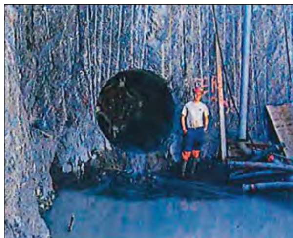
Figure 4 - Hesthaugen, Sandvika. Horizontal small tunnel, \phi 1850 mm, length 295 m, inclination = 0,07 % for leading surface/waste water away from the railway lines.
