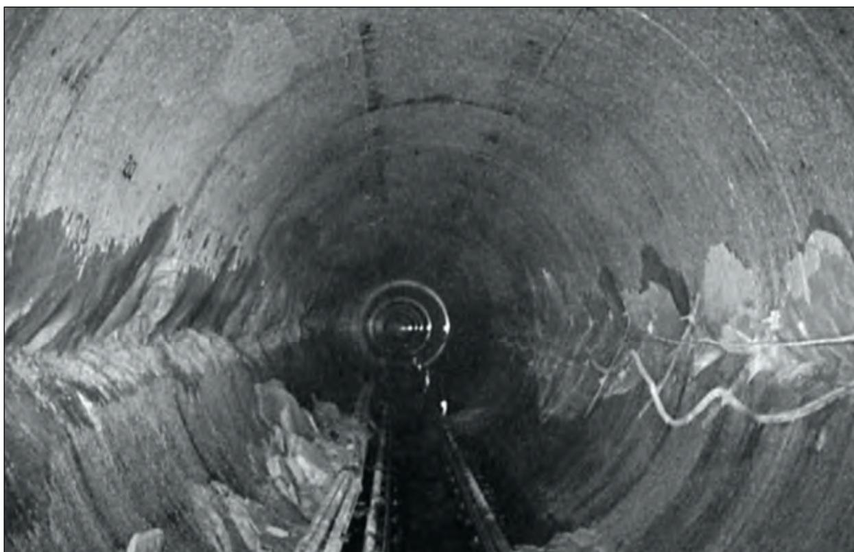
Figure 10. "Dog-earing" in sandstone due to high vertical stresses in the Delivery Tunnel in Lesotho
