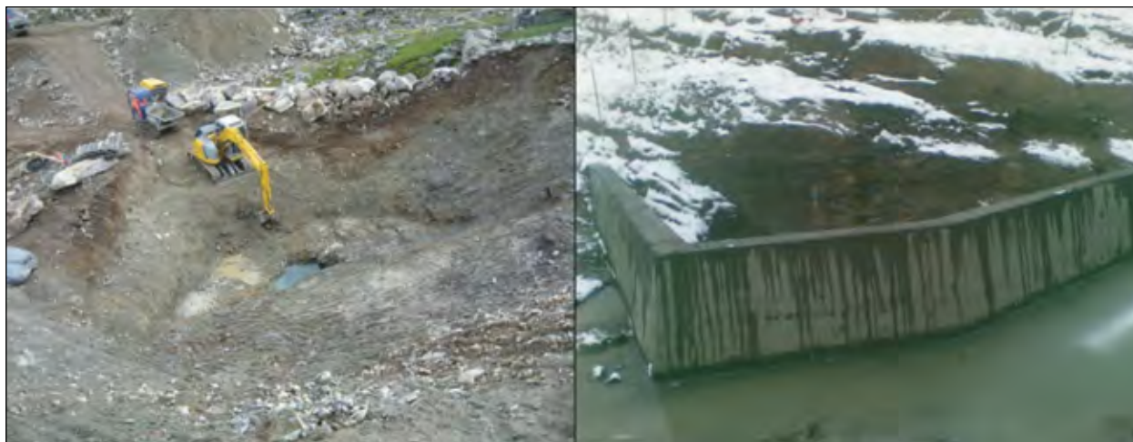
Fig. 4: Clearance and concrete protection wall at the sinkhole (Courtesy: Norsk Hydro).
