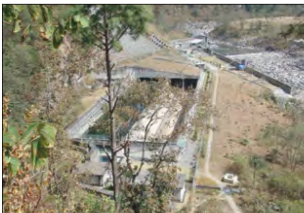
Figure 1: Khimti intake and desilting basin. The trap is incorporated at the end of the 7 km long headrace tunnel, just upstream of the pressure shaft.
