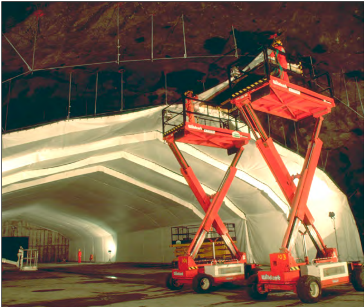
Figure 3 shows the installation of the WGTS in a rock cavern. From a final product at the far end to the on going installation work, using electrical driven lifts in the front. At the top of the picture we can see the rock bolts and the steel wire rope running between the rock bolts.
