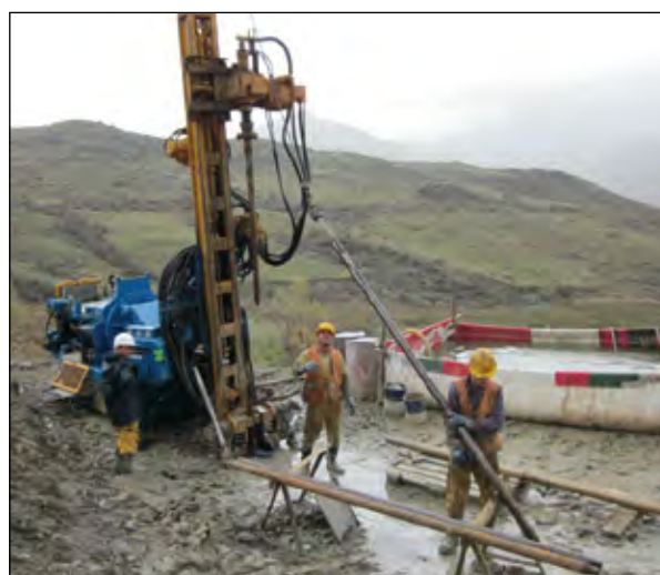
Figure 5: Core drilling in the Flysch
