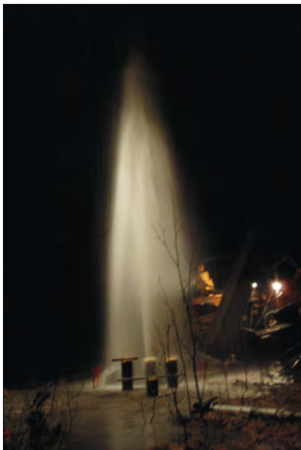
Figure 2 - Drilling into the water filled tunnel.
