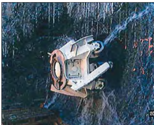
Figure 4 - Hesthaugen, Sandvika. Horizontal small tunnel, \phi 1850 mm, length 295 m, inclination = 0,07 % for leading surface/waste water away from the railway lines.
