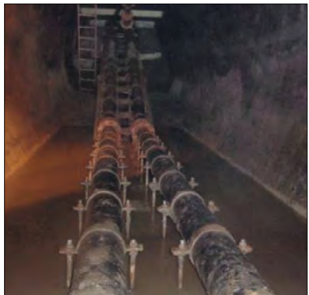
Figure 4: Tunnel desander and SediCon Sluices below the concrete slabs.
