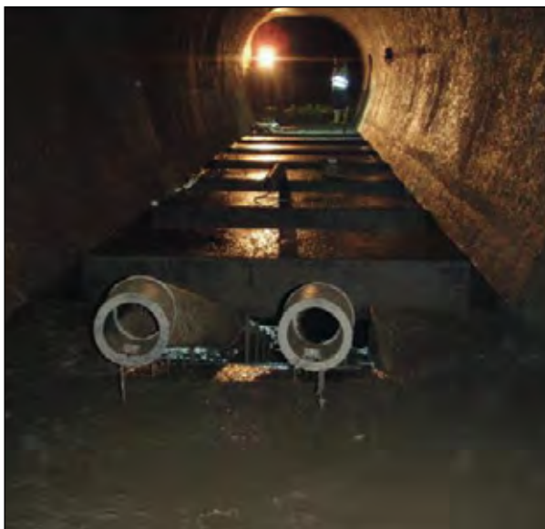
Figure 3: Tunnel desander above the concrete slabs. The upper ends of the SediCon Sluices are visible.
