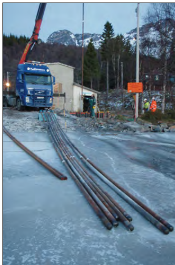
Figure 3 - Freezing pipes ready for installation. Gatehouse in the background.
