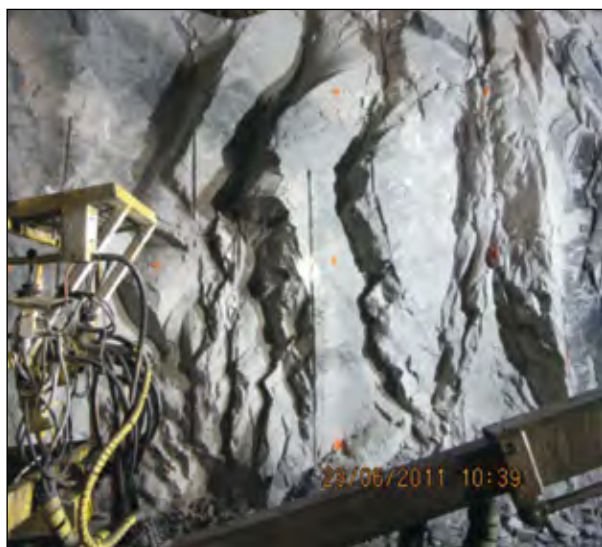
Figure 13: Shows secondary joint sets sub-parallel to the walls, that formed after blasting due to high rock stresses.
