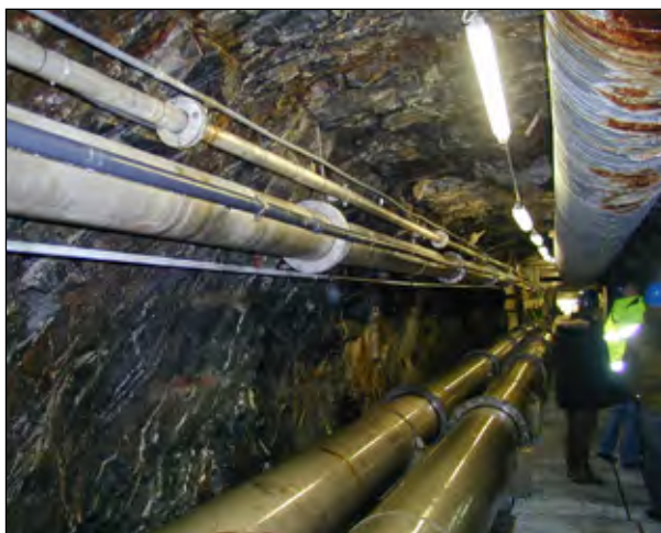
Figures 1 and 2: The picture to the left shows a typical situation in a pipe access tunnel where you have a wet and humid environment that gives corrosion problems to steel pipes and electrical equipment. To the right we see a picture of a complete different result after the installation of WGTS. The humidity is now under control and the life time for the assets has increased dramatically.
