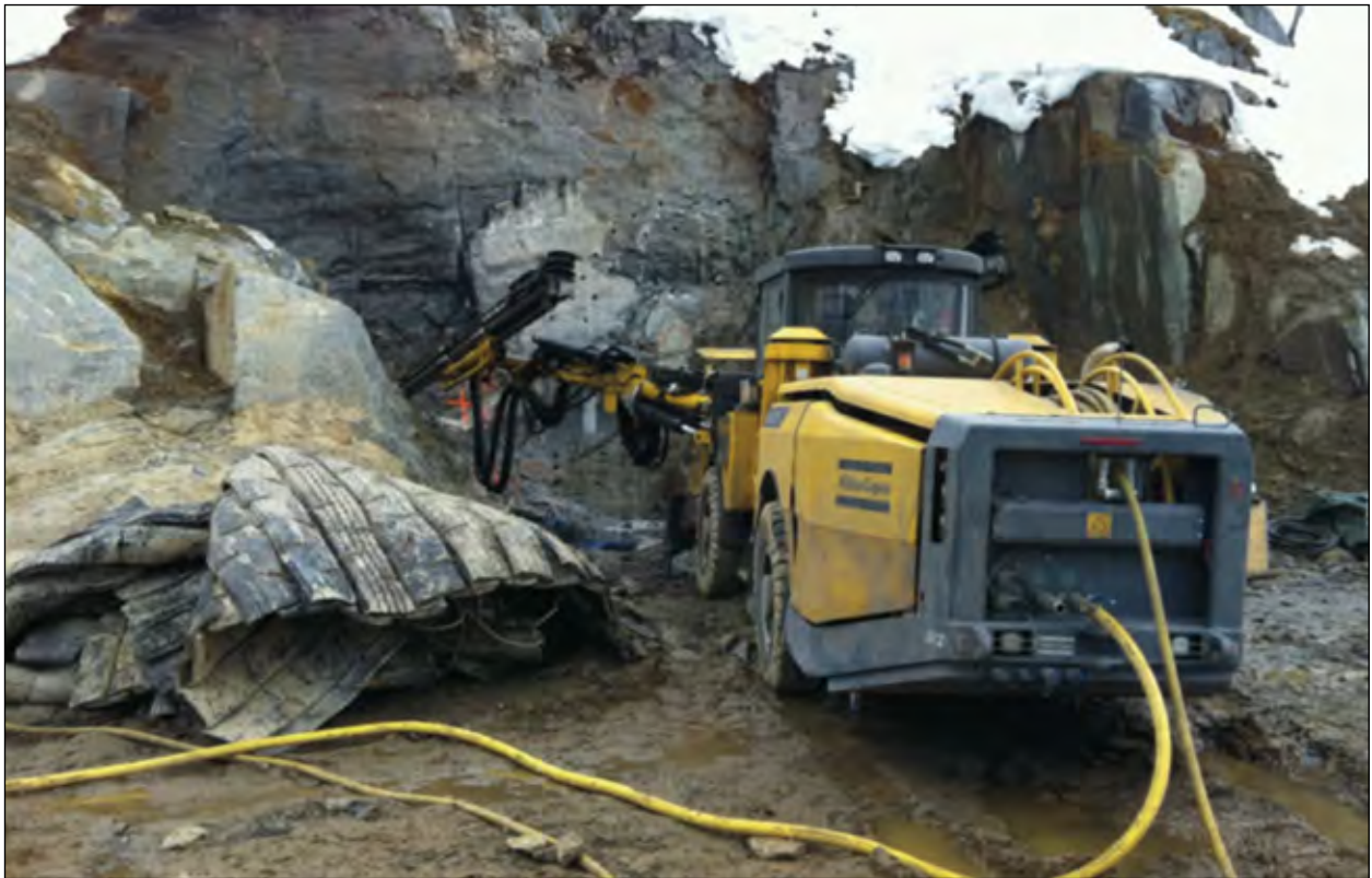
Figure 8 Securing and spiling
