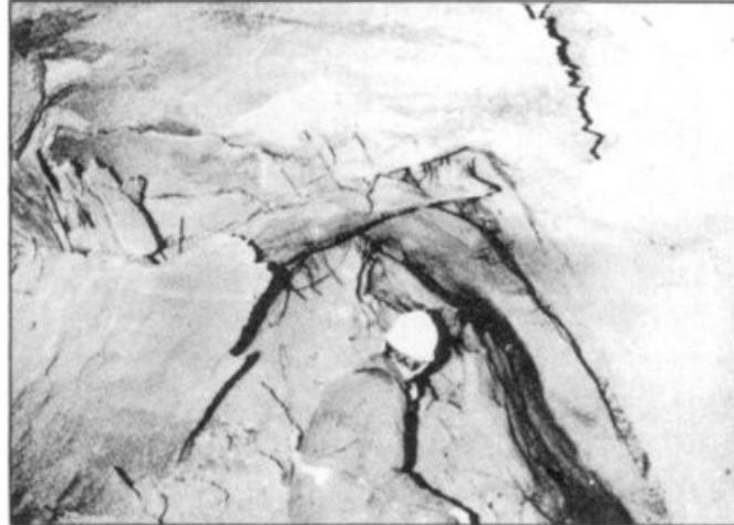
*Fig. 4. A total break down of a shotcrete lining in a water supply tunnel due to a gouge with swelling*
