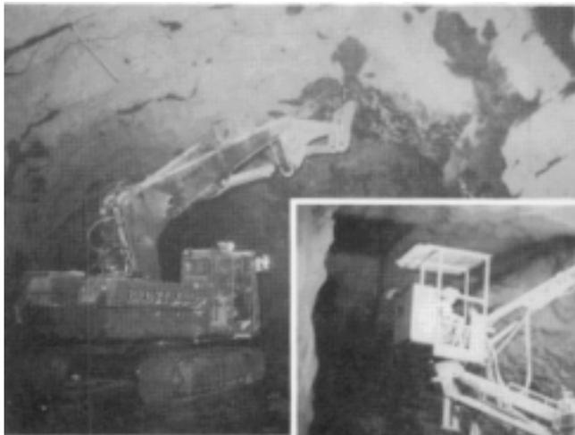
*Fig. 3. Modified backhoe excavator for mechanical scaling.*
