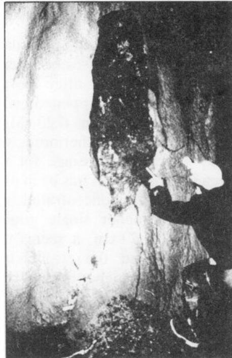
*Fig. 3. Failure due to swelling clay in water supply tunnel.*
