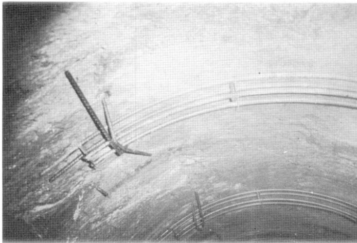
*Fig. 10 Tunnel wall with rebar steel basket for shotcreting of ribs*
