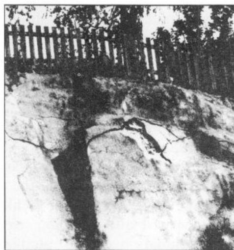
*Fig. 2. Shotcrete failure in an open cutting due to frost burst.*
