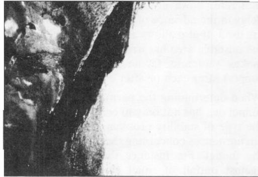
*Fig. 1. Failure due to joint plane and frost action in a tunnel.*
