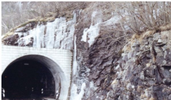
The left side portal is well designed, whereas the right side structure gives the impression of a simple makeshift set up. Both structures, however, is designed to stop incidental blockfall of ice and rocks, water leakages and landslides at the entrance of the tunnel
