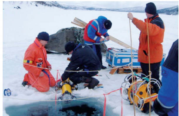
The partly collapsed tunnel between the lakes Bleikvatn and Røssvatn was not accessible and subsea ROV vessels were used for inspection
