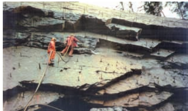
Rock support outside new access. Also from the VEAS facilities.
