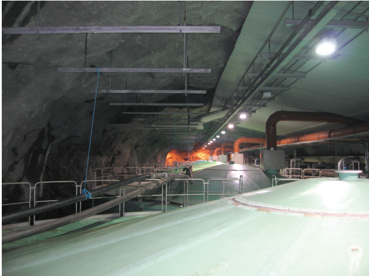
From waste water treatment plant near Oslo with limited access for repair or improvement of rock support.
