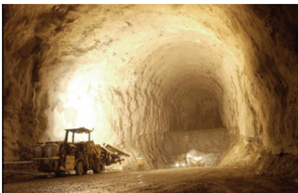
Rock cavern for oil and gas storage
