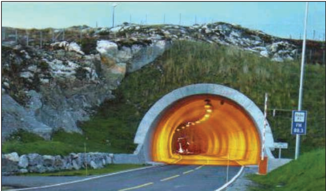
Fig.1 Portal of a Tunnel showing the barrier for closing the tunnel
