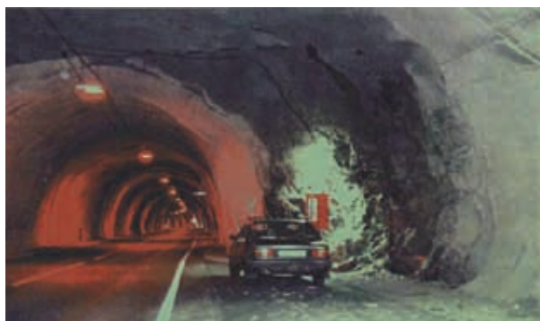
Fig. 1: Typical situation inside a Norwegian low traffic tunnel
