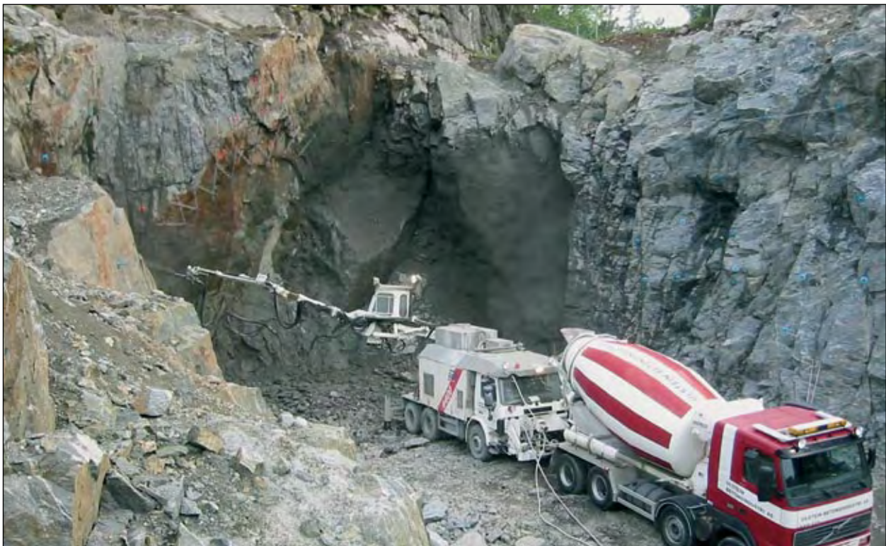
Support of opening with sprayed concrete.
