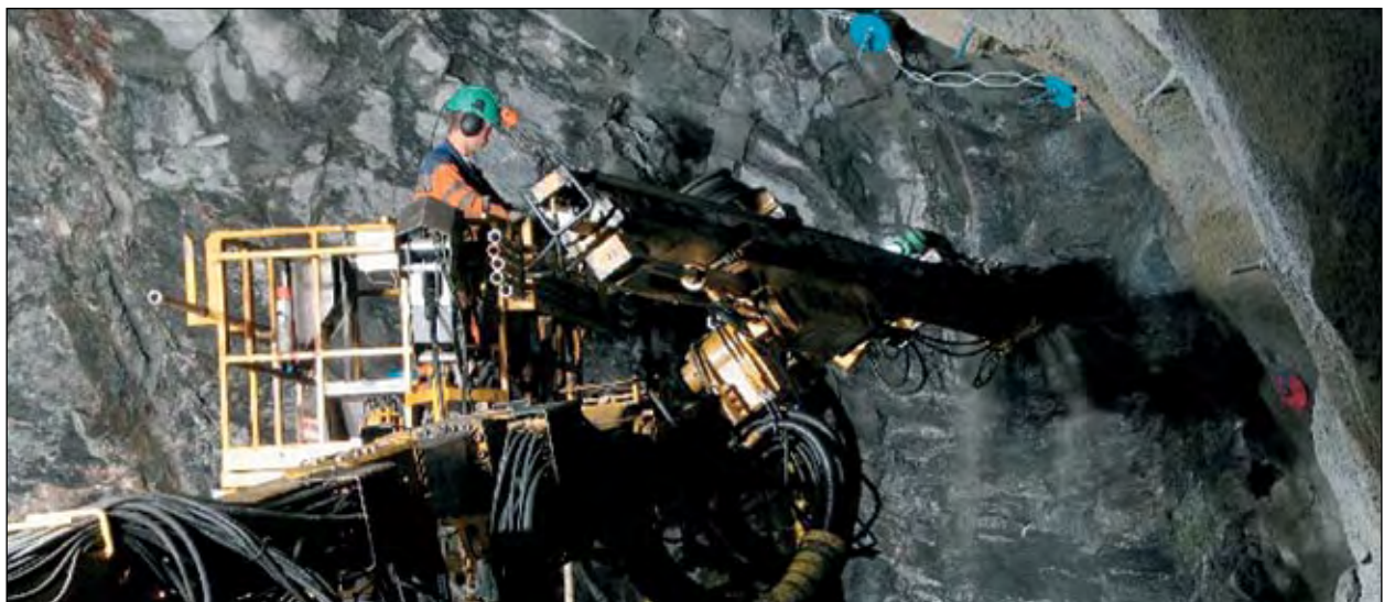
Exploratory drilling, changing of drill rod.
