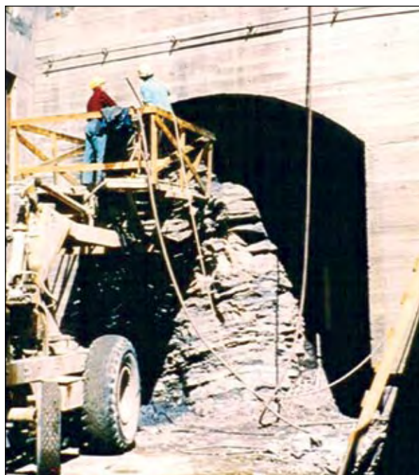
Fig. 1 shows the preparations for the main entrance tunnel to a telecommunication facility in rock.
