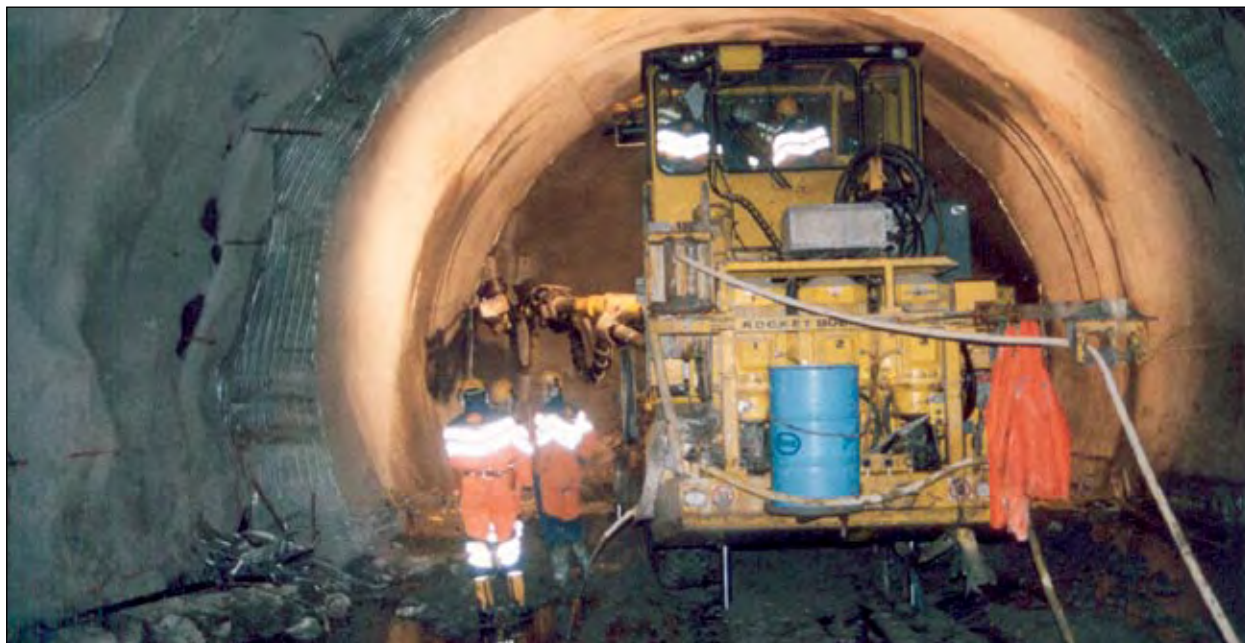
Figure 8. Drill and blast excavation in difficult rock mass conditions in the Frøya tunnel. Extensive shotcreting and concrete lining were required.
