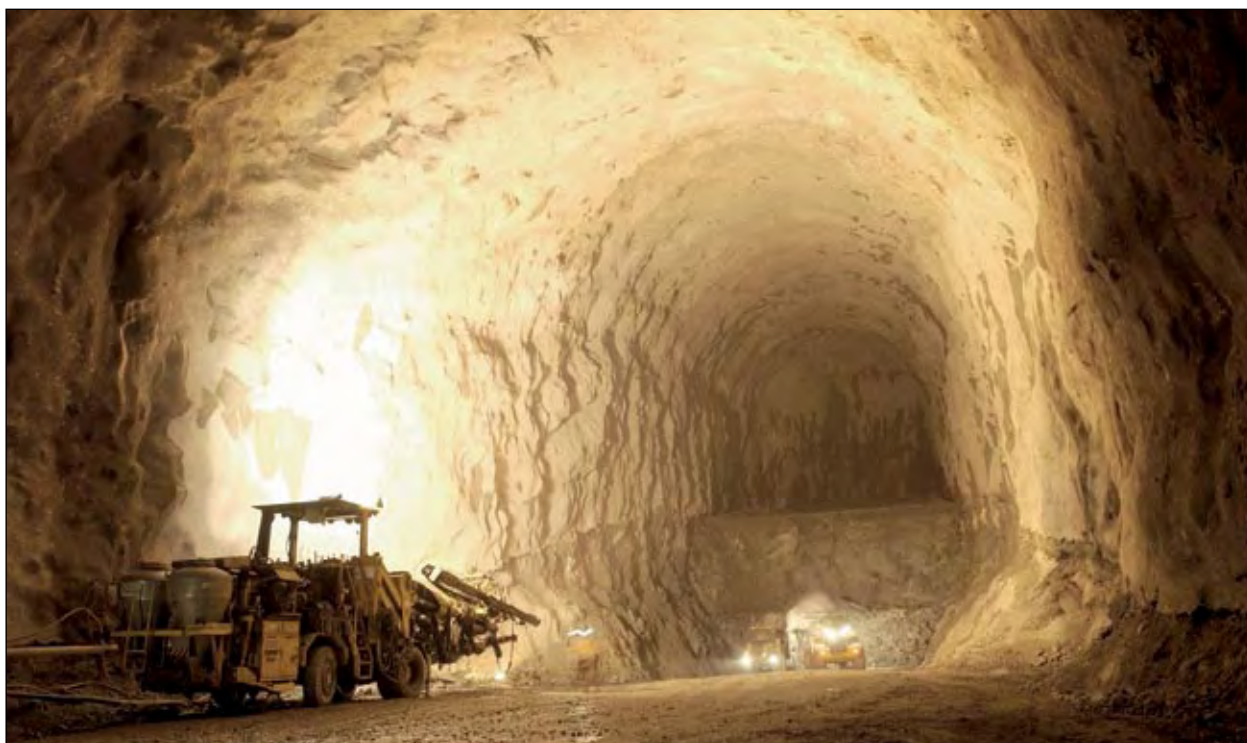
Rock cavern for storage of low temperature gas at Mongstad refinery, north of Bergen
