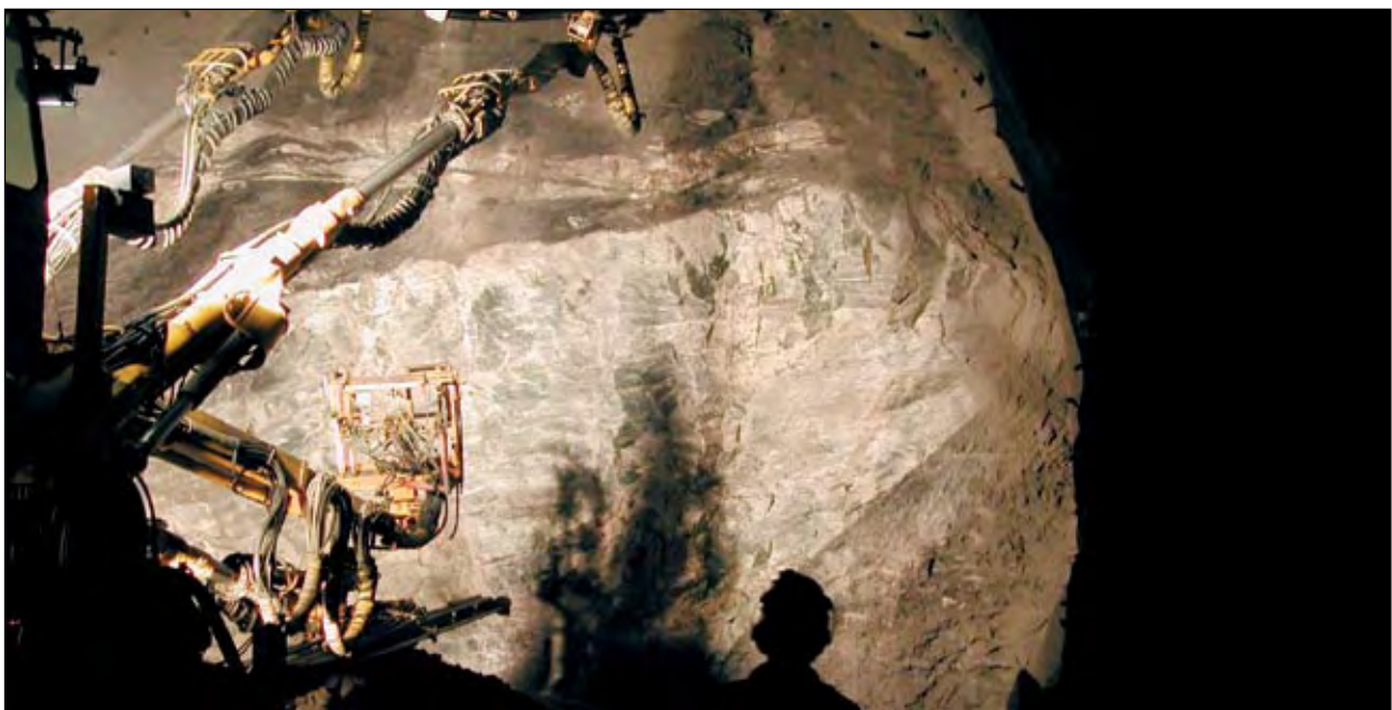
Drilling at tunnel face.
