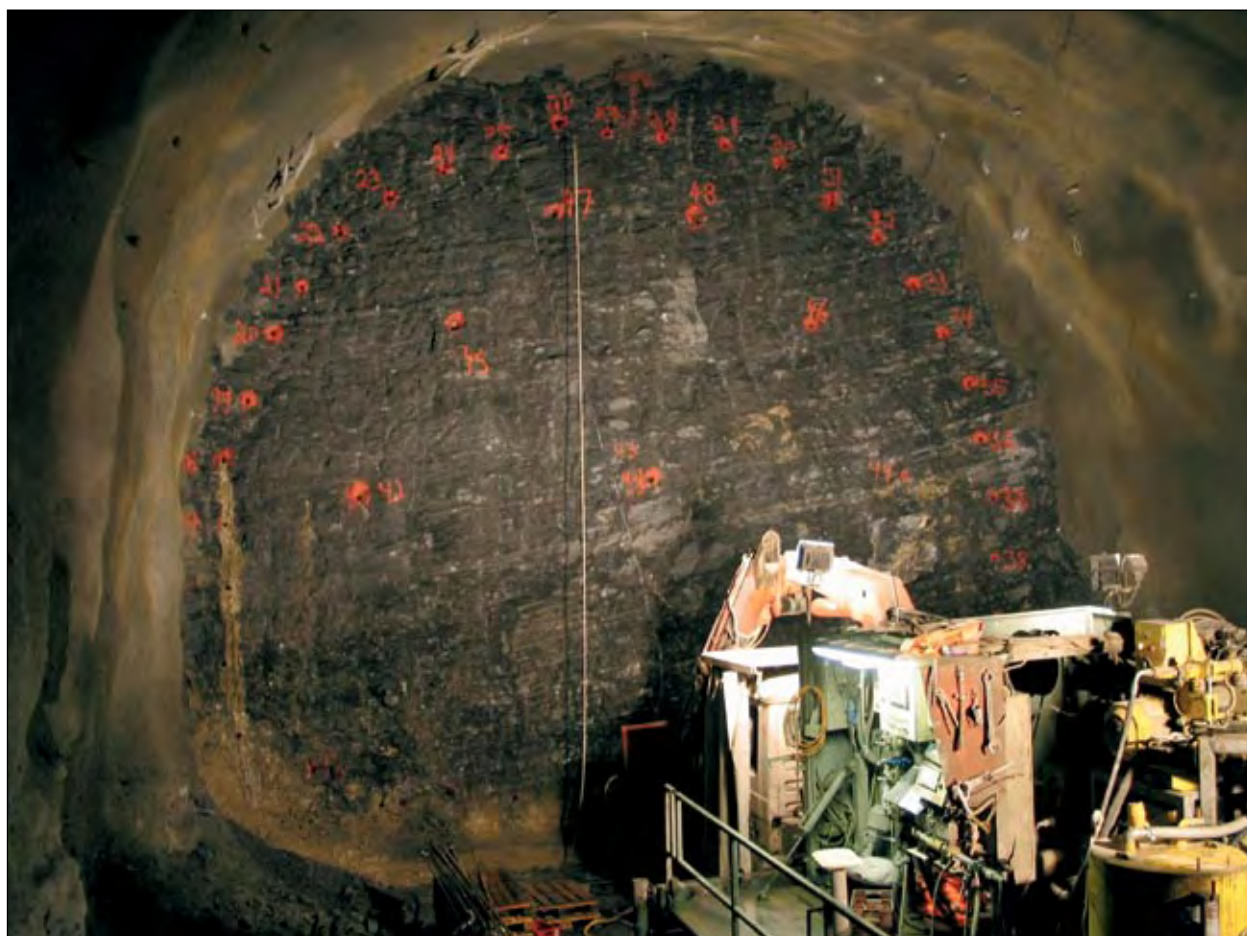
Figure 2 The Tanum tunnel (Jong-Asker railway). Markings of injection holes in the tunnel work face.
