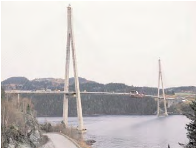
The Skarnsundet Bridge is a 1,010 m long cable stayed bridge with 12 spans. The main span is 530 m long and the A-towers are 152 m high. Veidekke was honoured by the National Association of Architects for this project.
