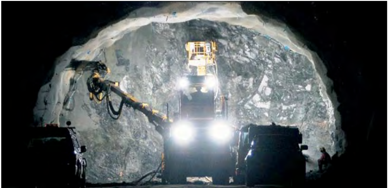
Exploratory drilling at profile 1614.
