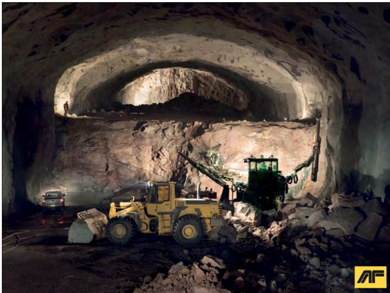
Figure 9: Bench excavation by horizontal drilling and blasting. The top gallery is completed.. Photo: C. .F. Wesenberg.
