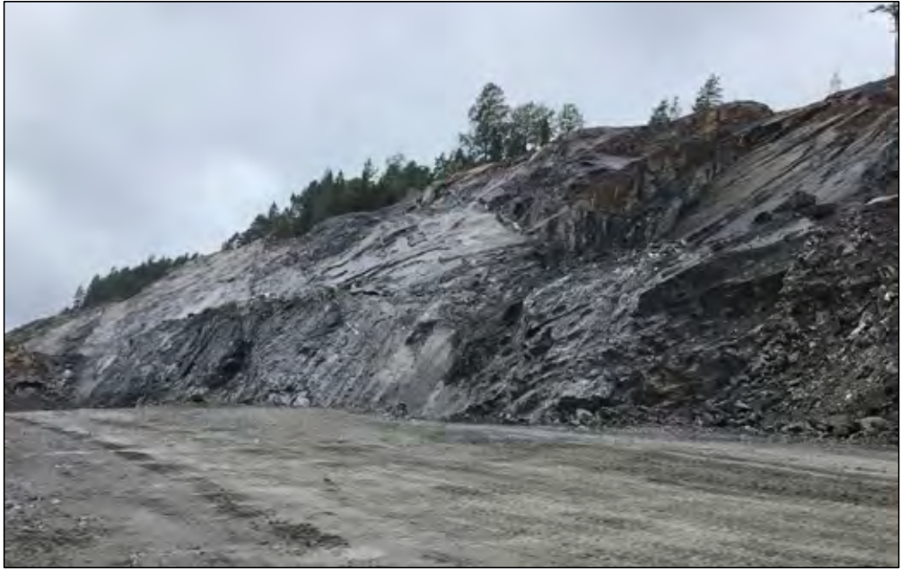
Fig 2 A portion of 15330-16360R showing surface of pervious planar slide along the foliation surface in the top right corner.
