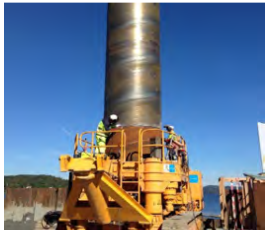
Figur 13: RDM 2000 Casing Rotator
