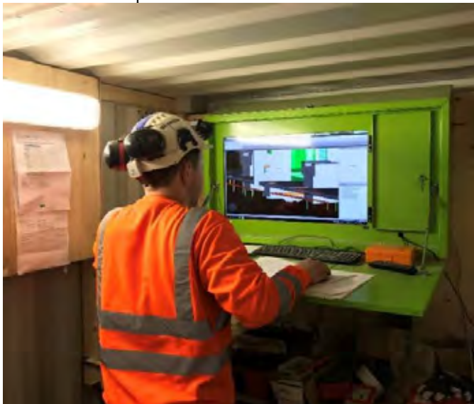
Figur 9: BIM-kiosk (grønn) inne i container
