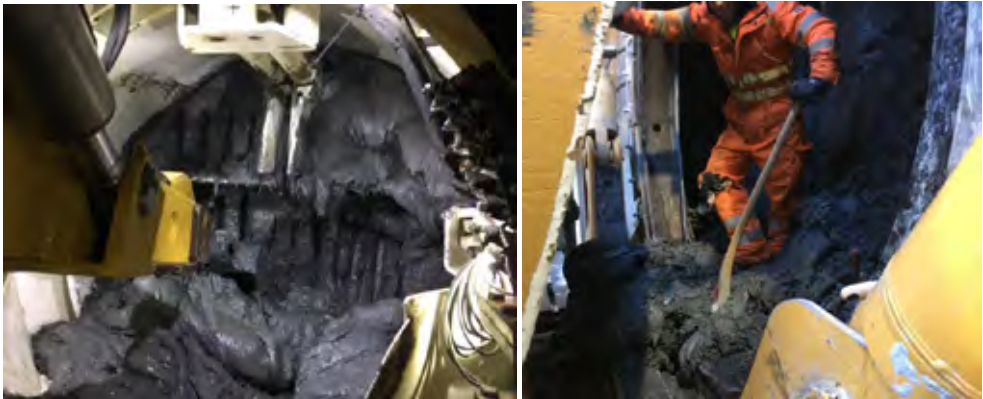
Figur 21: Graving i front
