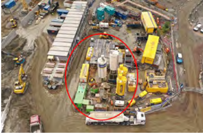
Fig.9: Site setup: mixing station for 2 jet grouting units (red circle) and backflow treatment plant, on the right side the single entrance to the site can be seen
