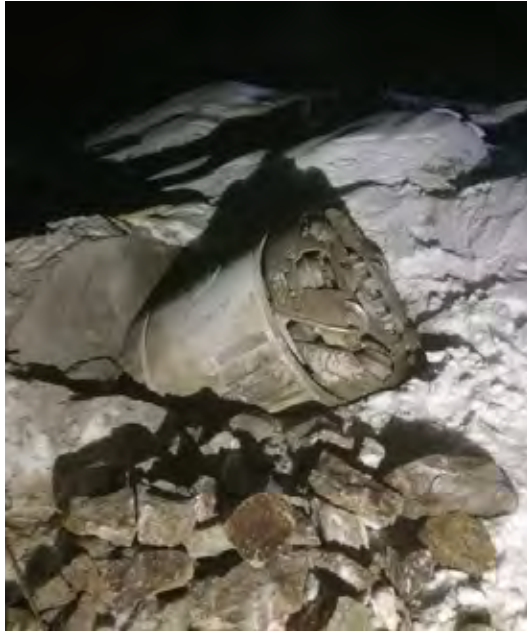
Figure 7 Breakthrough at Holen (Photo; Hardanger Maskin AS)
