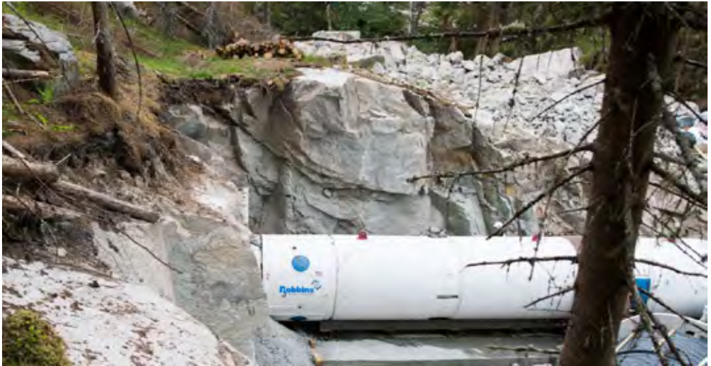
Figure 6 TBM at Holen HEP (Photo: Endre Hilleren)
