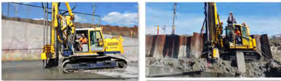
Fig.10: Left is the double axis jet grouting rig and right the single axis rig executing the soil improvement works
