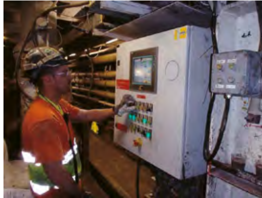
Photo 9 Grouter on TBM back-up operating the HÄNY batching plant during the construction of an barrier
