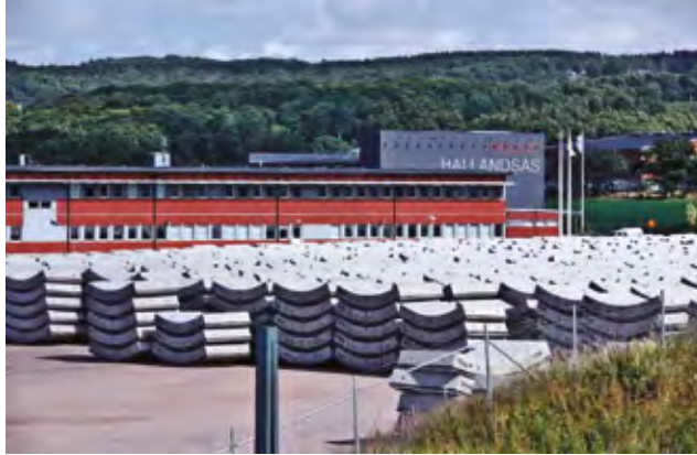
Photo 6 Segment storage area with Main Office (to the left side) and Hallandsås Tunnel exhibition hall (to the right side)
