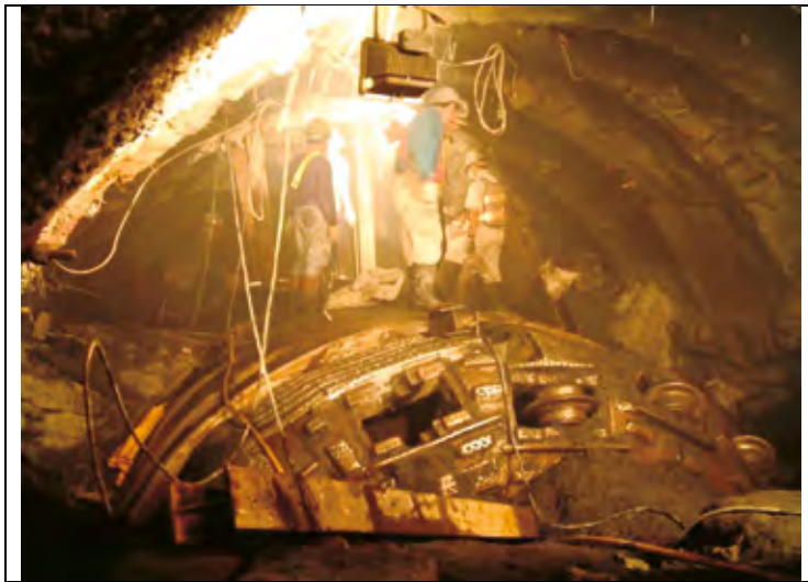
Figure 20 A pilot tunnel for drainage and pre-injection across to the main tunnels, as used successfully at the Channel Tunnels in chalk-marl, was not successful at the Pinglin Tunnel project in Taiwan, due to numerous cutter-head blockages and need for side-access drifts (at least 13 times). In addition the contractor had great difficulty even drilling stable holes for pre-injection, due to the intensely jointed, sheared and clay-coated joints and slickensides in the very hard meta-sandstones. Photo: Chris Fong.
