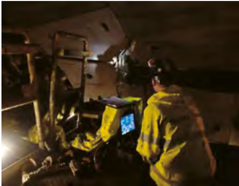
Photo 8 Driller operating a drill rig on the TBM during an Probe Drilling exercise
