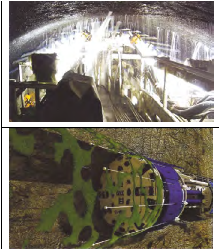
Figure 29 Robbins (D.Wallis, 2012) illustrations of the need for pre-injection and its solution with the ACT illustrated in Figure 28. Water is a remarkably adverse ‘partner’ in tunnelling, but its unwanted presence can be severely curtailed if pre-injection is an accepted measure. This measure is however ineffective if too low injection pressures are used. At least 50% of the injection pressure at the pump has been lost, just 1m away from each injection borehole. When flow stops, pressure must not be maintained. The job is complete. Barton (2011/2012).
