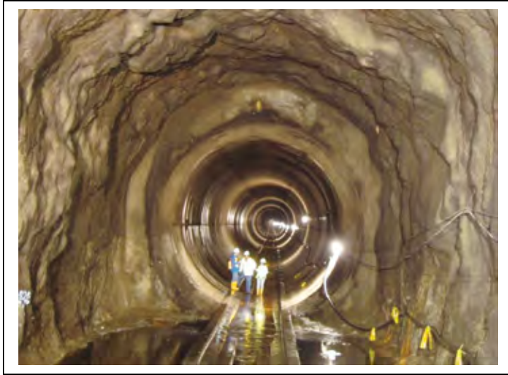
Figure 25 A double shield TBM used to drive a 10 km long headrace tunnel in Ecuador, where inspection during second emptying was led by the writer, on behalf of contractor Odebrecht. This project was unusual because the PC-element lining had been used in thirteen specific stretches of bad ground, where the advantages of 'ready-made' support and push-off-liner thrust could be fully utilized if no gripper operation was possible. A serious fault zone nevertheless stopped the machine for several months in one of the thirteen locations. Photo: Dr. Nghia Trinh. Note that wedges and small blocks that had fallen from some locations in the many unlined kilometers were not transported, even by 2.5 m/s water flows. The so-called 'rock trap' contained only sand and silt and some floating pumice 'pebbles' from upstream. The 'zero velocity' boundary layer ensures transport of nothing larger than rounded, few millimeter size particles. The hydraulic boundary layer phenomenon therefore indirectly provides us cheap renewable power in Norway and wherever 'nominally unlined' hydropower tunnels are used. There are 3,500 km in Norway, 250 km driven by TBM.
