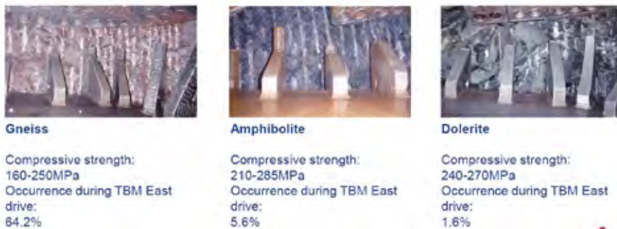
Figure 3 TBM faces showing Gneiss, Amphibolites and Dolerite
