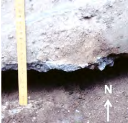
Figur 11: Fundament akse 23/AL.
