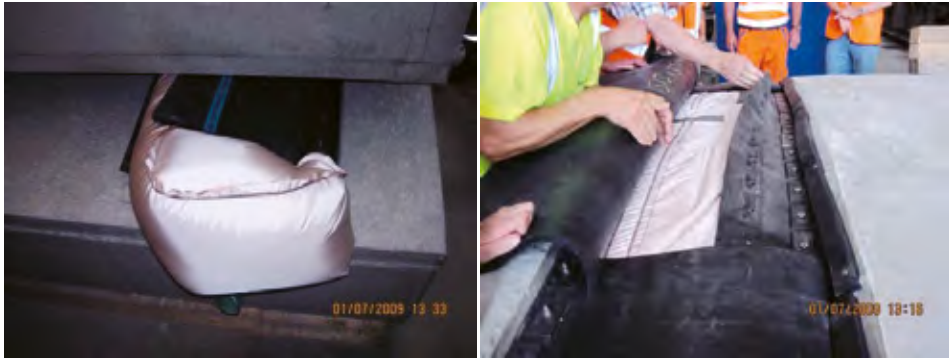
Photo 10 External bag attached to a prefab concrete segment
