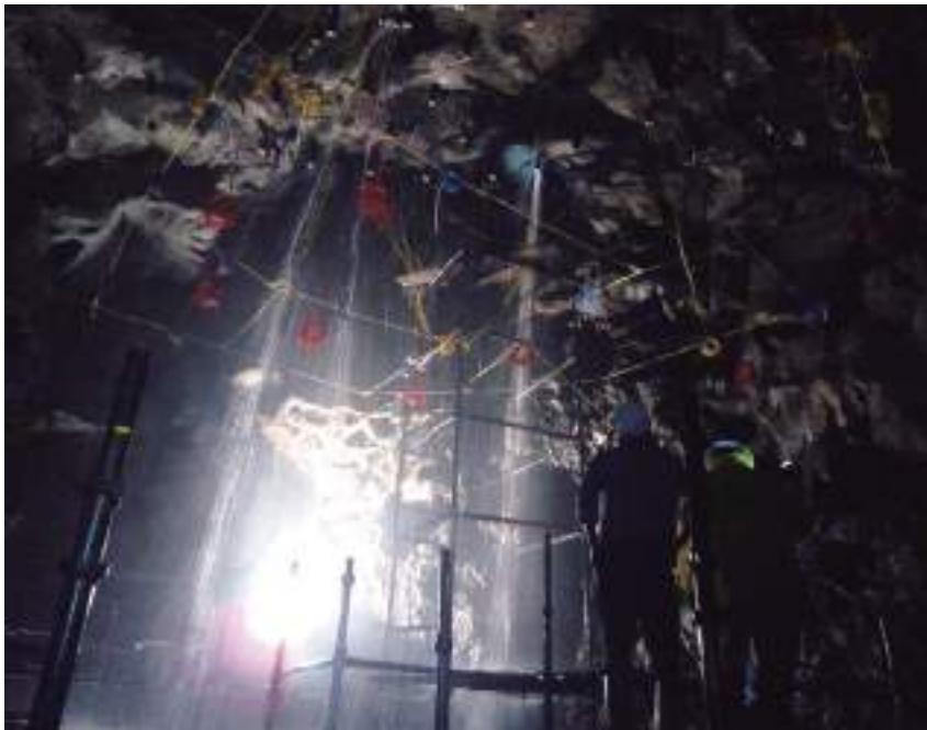
Figure 8 Intense leakage occurring after completed charging.
