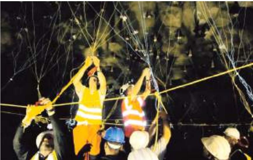
Figure 7 Tie in of nonelectric detonators.
