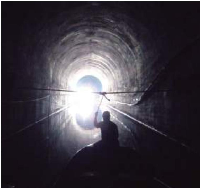
Figure 10 Access by boat across the spoil trap, for final tie in of electronic detonation system.
