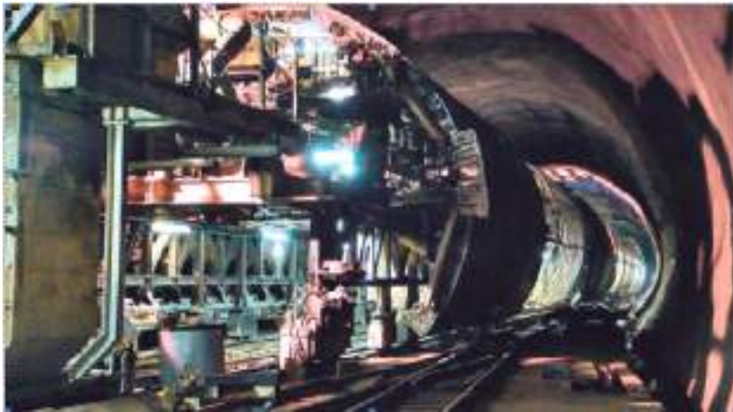
Figure 6: The east “worm” near the Faïdo MFS; preceding and trailing shuttering systems, “elbow joint”
