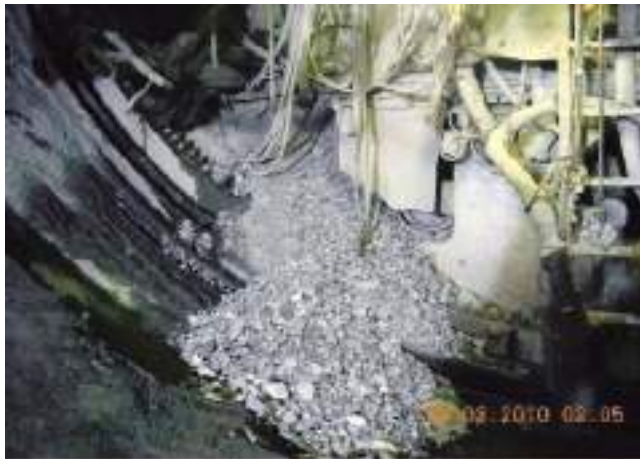
Figure 16: Standstill of the West Tube TBM
