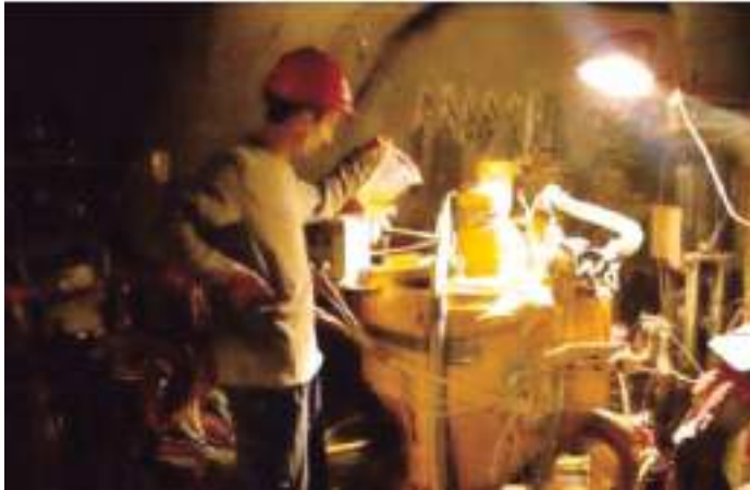
Figure 17: Grouting work from the niche
