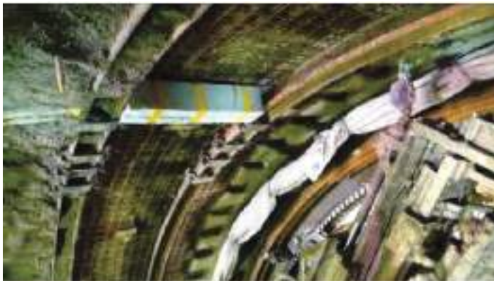
Figure 11: Longitudinal convergence slot with Styrofoam insert
