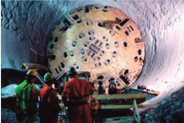
Figure 9: Maintenance of the cutter head of the western TBM during the Christmas/New Year break, 2010/2011
