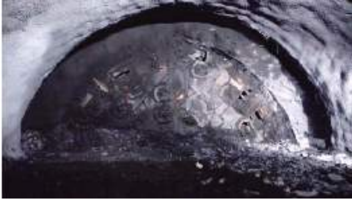
Figure 18: Successful restart of the West Tube TBM
