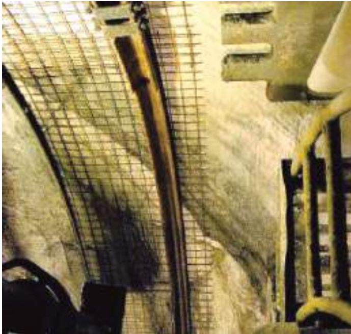
Figure 15: Eastern TBM in the Piora Syncline
