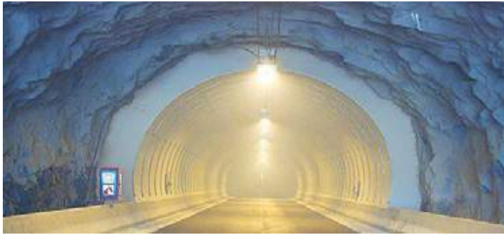
Figur 8. WG Tunnelhvelv T100
