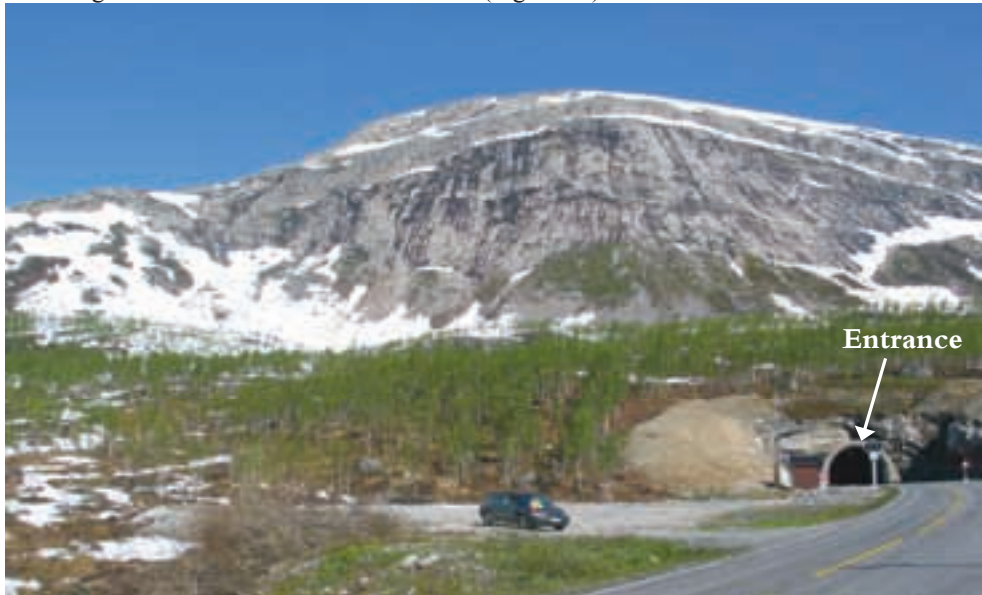
Figure 10 Photo of the entrance to the Kobbskaret tunnel
