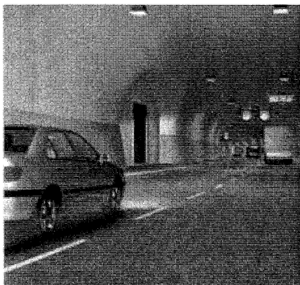
It will be possible to use the access tunnel as an escape route through the fire doors built every one hundred metres.
