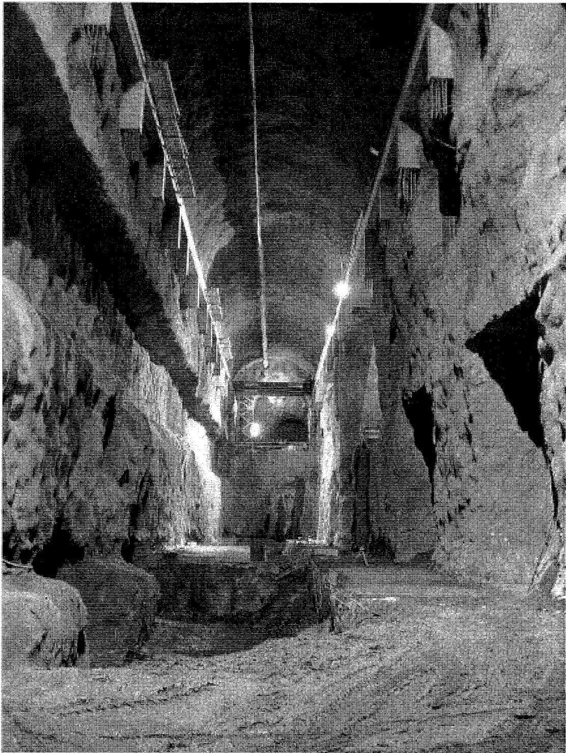
Figure 23. Successfully completed excavation and rock support of the powerhouse cavern, in early December 2004
