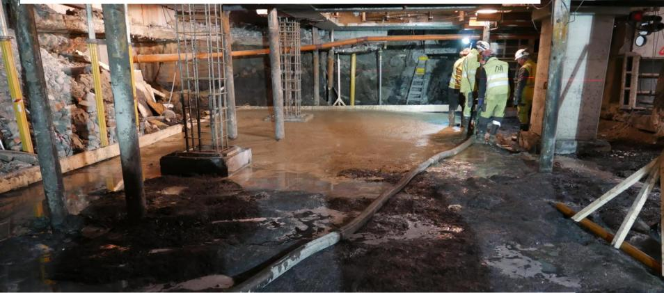
Alum shale surface impregnated with NaOH/KOH emusion before covering with concrete, membrane and a new layer concrete to make up the basement floor
