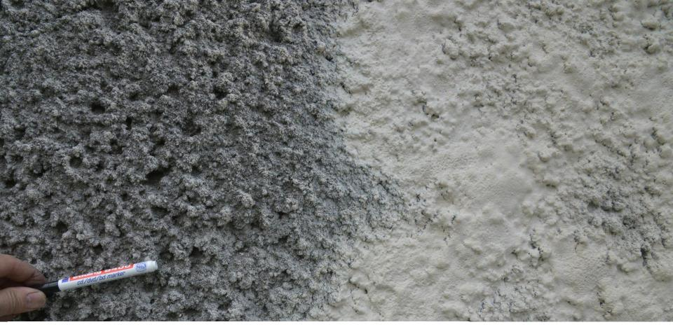
Shotcrete surface must be smoothend. The surface in the picture is too coarse
