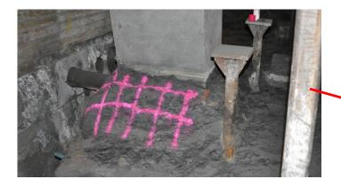
Foundation reinforcement with epoxy injected into cracks in the alum shale
