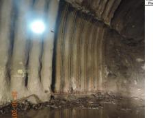
Pre-fabricated steel arches, pre-bolting, CT-bolts
