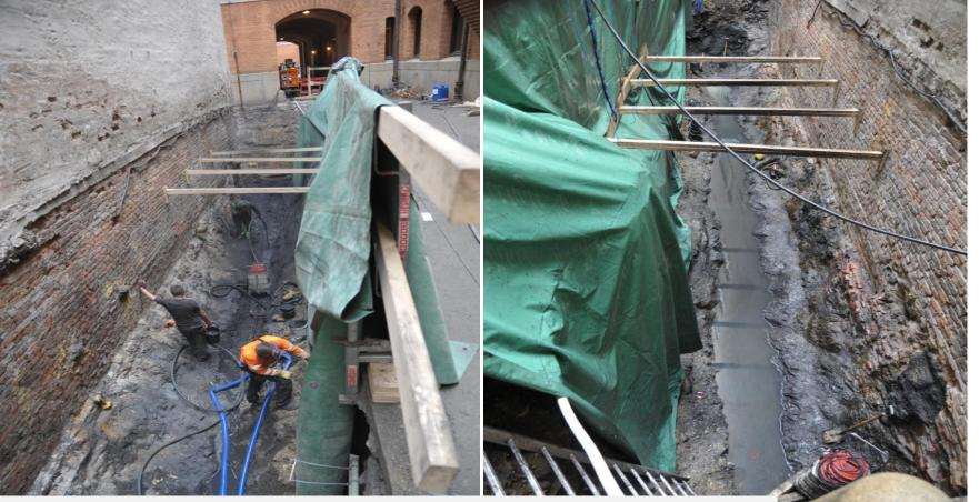
Chemical grout – colloidal silika, viscosity like water. Long reaction time (> 12 hours) to secure optimal infiltration along the waterway. Gravity driven infiltration of colloidal silika
