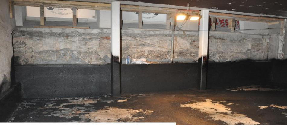
Asphalt-bitumen water based membrane High stretching capacity, Low strength Primarily used on horisontal surfaces Effective sealing, large areas, specialized equipment and personell White spotted areas are excess water form the hardening process
