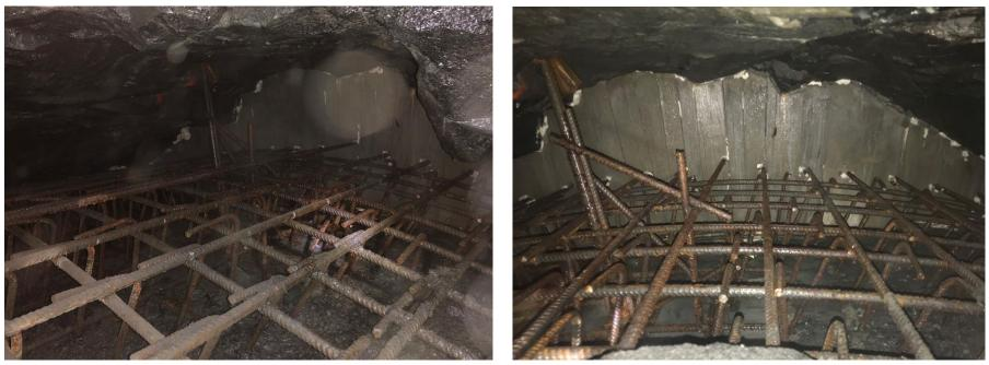
Concrete missing above the roof of the sewage tunnel; 3,5 m in the direction of the TBM drive and maximum width of 5 m
