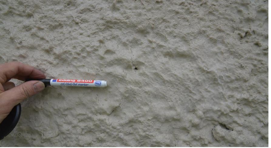
Too thick layers will cause cracking
