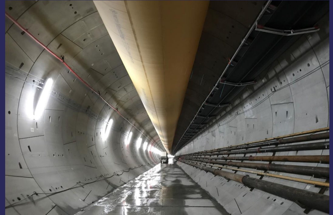
Photo from the Follo Line Tunnel
