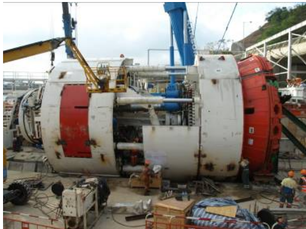
26-Feb-2009 – Forward Thrusters Testing
