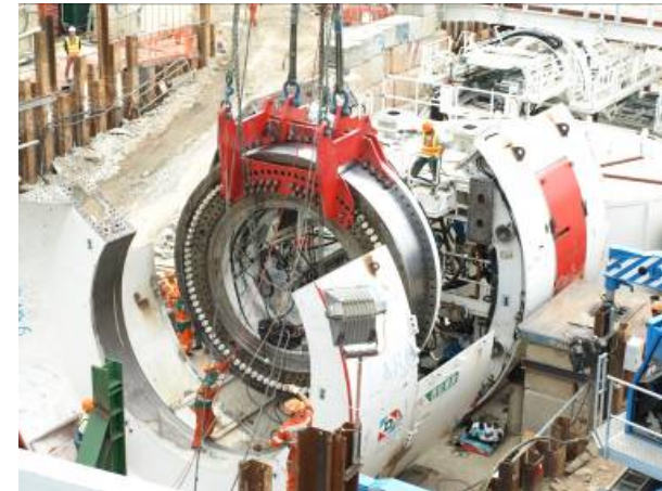
18-Feb-2009 Main Bearing Installation
