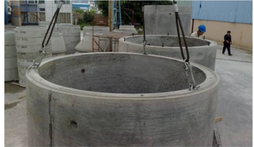
Install ring clutch to lifting lug
