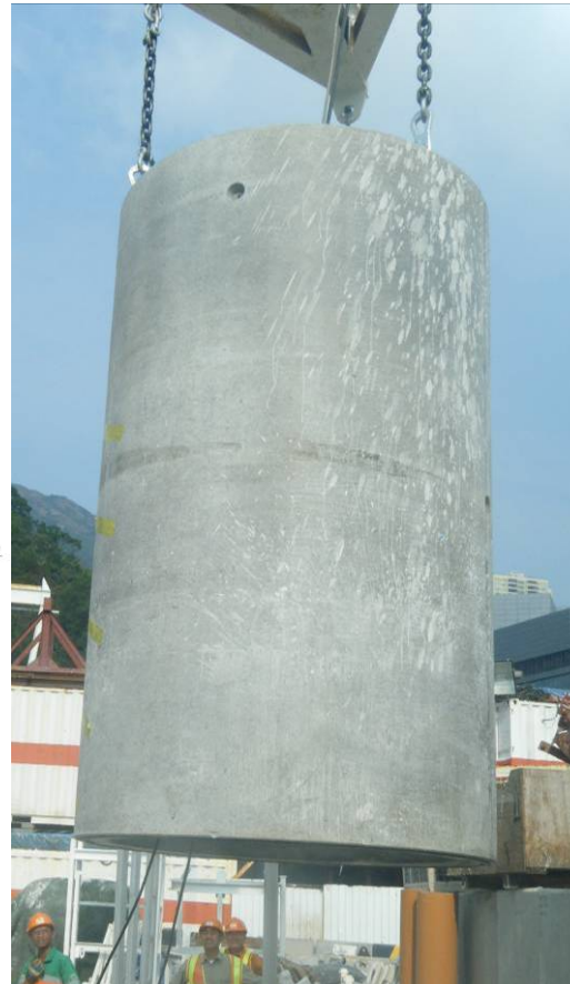
Lay shear shape into centering cone recess at upper face
