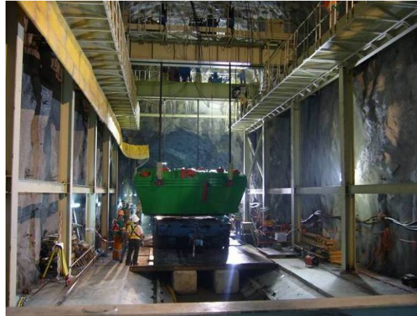
23-March-2009 – Unloading Cutterhead
