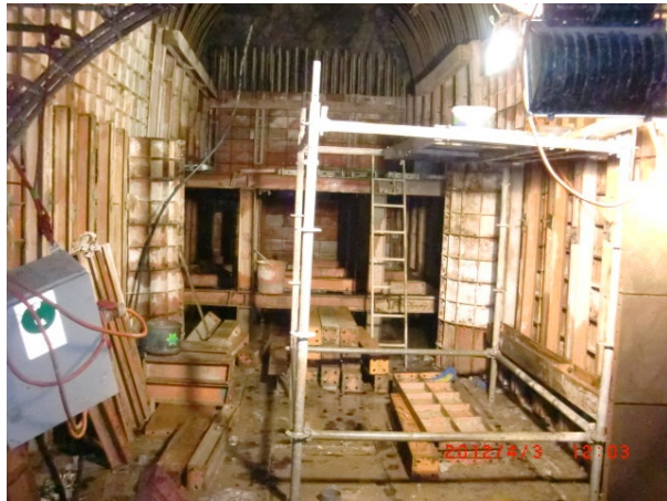
Formwork Erection at Stilling Chamber
