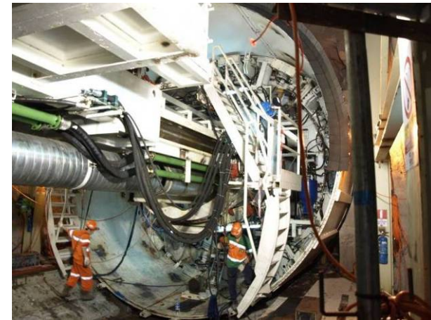
29-Apr-2009 – TBM Shield in Start Position Start Back Up Assembly
