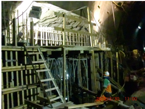
Formwork Erection at Adit / Main Tunnel Junction
