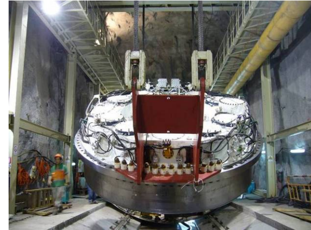
31-Mar-2009 – Lifting Main Bearing for Installation
