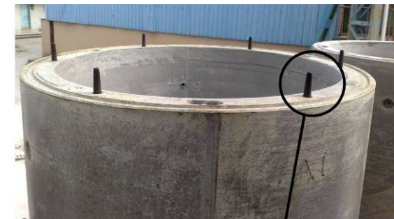
Lay shear shape into centering cone recess at upper face
