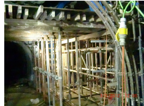
Formwork Erection at Turning Bay
