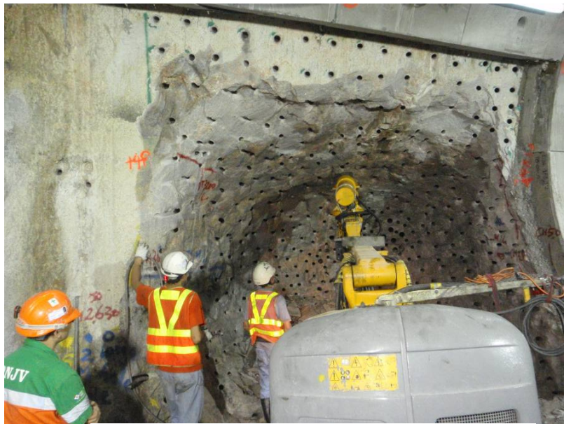
Mechanical Excavation
