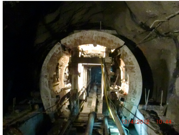
Typical Lining Formwork
