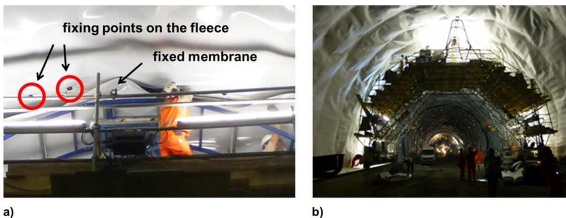
**Figure 5. Sealing membrane: (a) welding points on the fleece; (b) special scaffold for the installation.**
