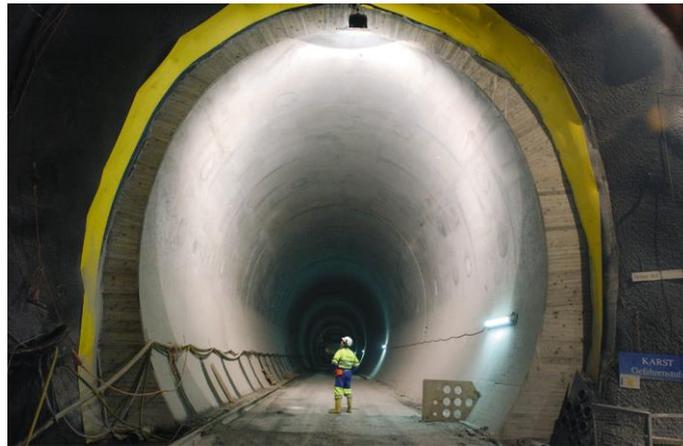
**Figure 9: Inner lining of the Lötschberg Base Tunnel (Switzerland) [10].**
