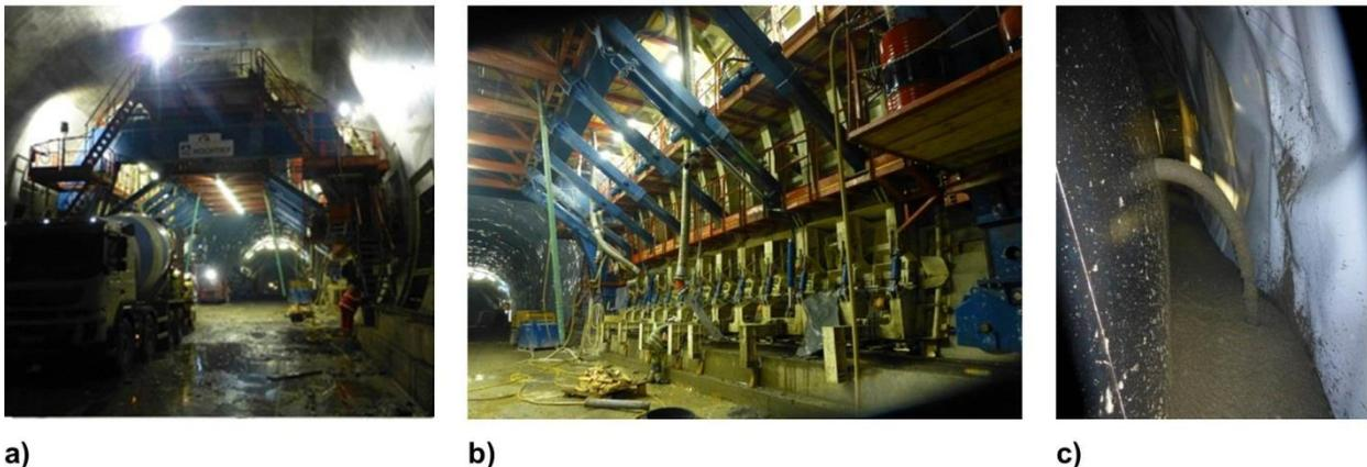
**Figure 7. (a) Formwork; (b) steel structure of the formwork; (c) concreting (left: formwork, right; sealing membrane).**
